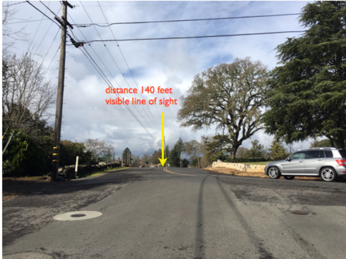
Visible Line of Sight is 140 feet from the Kreuzer Lane stop sign (at stop line). In image above, a car can be seen in the far distance, but will shortly disappear into the dip in the road and then reappear at 140 feet.
