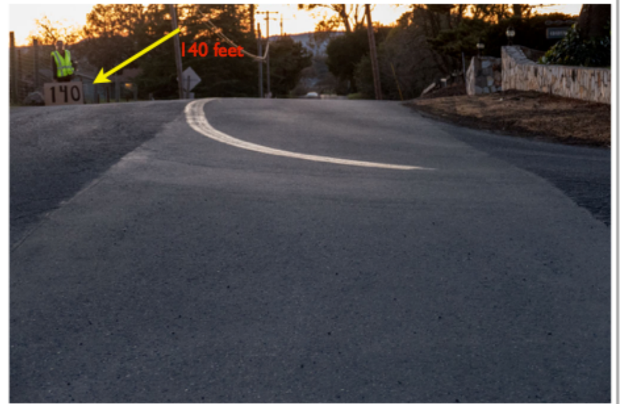
Visible Line of Sight is 140 feet from the Kreuzer Lane stop sign (at stop line). In image above, a car can be seen in the far distance, but will shortly disappear into the dip in the road and then reappear at 140 feet.
