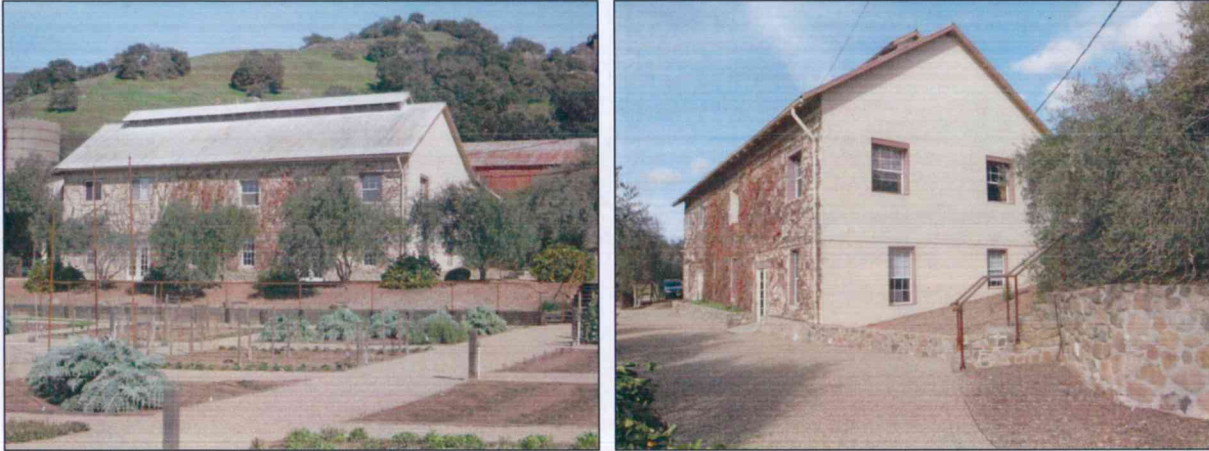
Figures 9 and 10. Left image shows the west elevation with corrugated monitor roof and windows inserted in the building wall. Right image shows the south and west elevations, with windows and doors inserted into the building walls. Compare this image to the historic view of the south elevation, shown on Figure 6.
