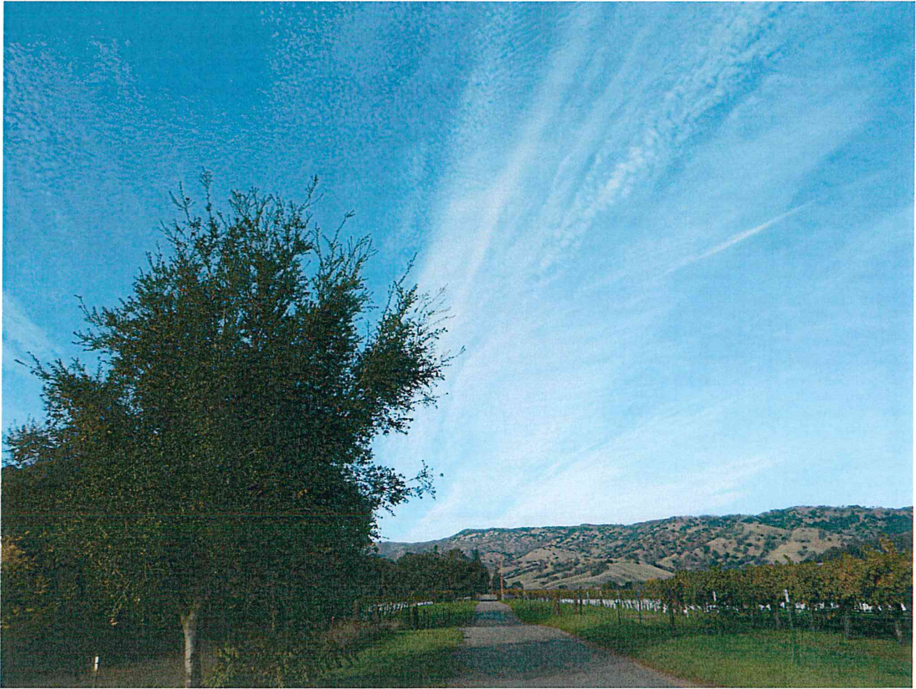
View of existing private common drive (Grapevine Lane) at approximate station 34+00 where the driveway will be fully improved to 22 feet wide.
