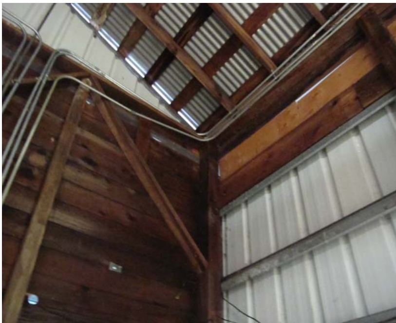
Figure 4. Interior showing framing and remnant of wood siding.
