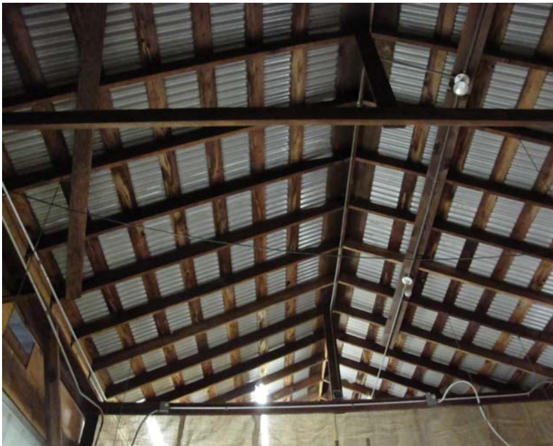
Figure 3. Interior showing roof framing.
