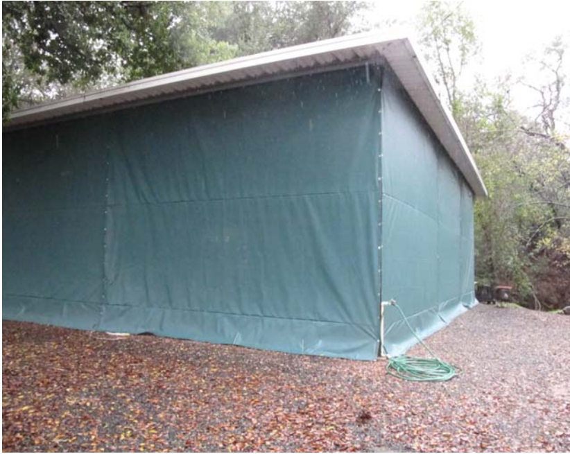
Figure 1. Oblique view of the front of the drying shed
