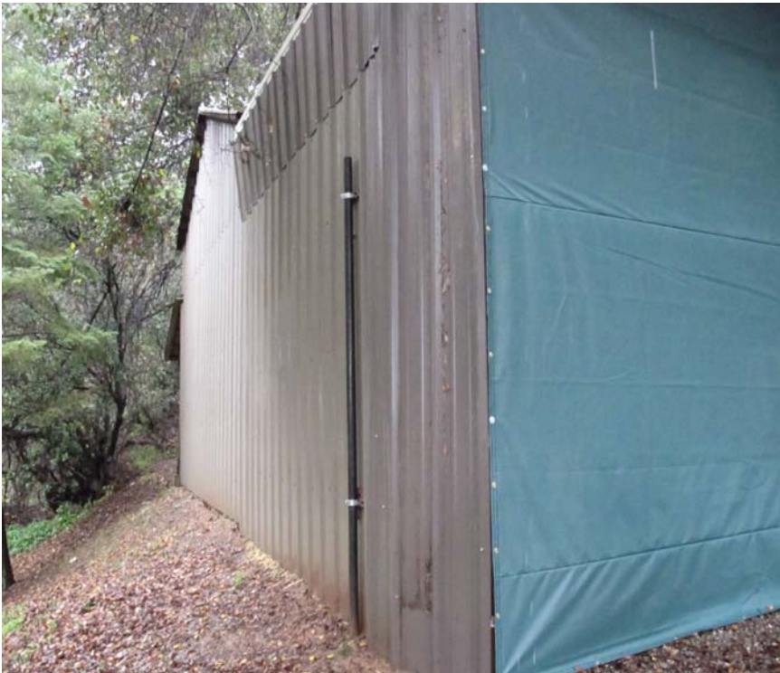
Figure 2. Oblique view of sides of the drying shed.
