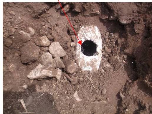
Leach line free of obstructions.
