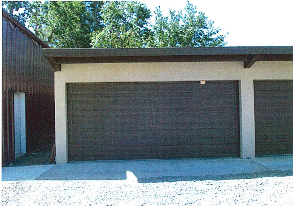
Photograph 29: Southerly panoramic view of existing structure. June 18, 2014
