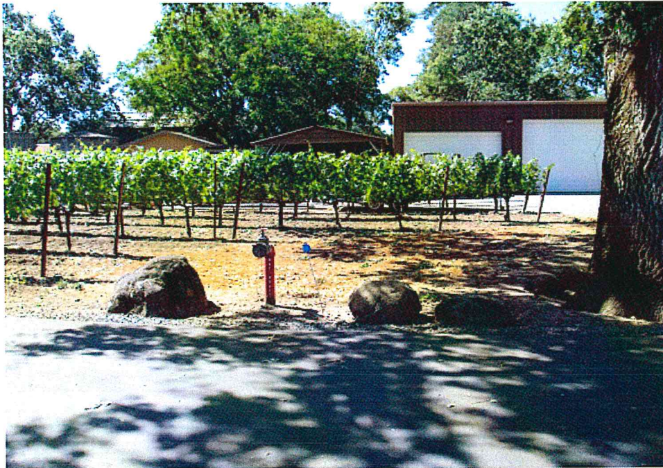
Photograph 31: Southwesterly view of existing wharf hydrant (1 of 2). June 18, 2014
