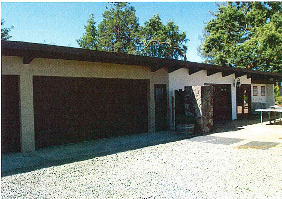
Photograph 30: Southwesterly panoramic view of existing structures. June 18, 2014
