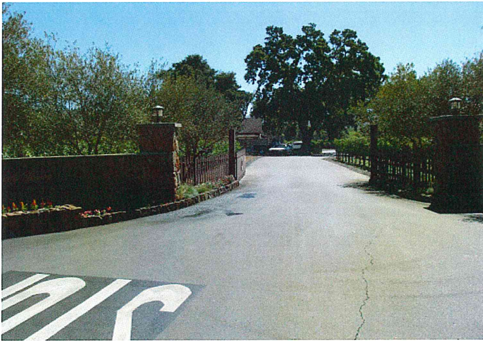
Photograph 14: Easterly panoramic view of existing driveway. June 18, 2014
