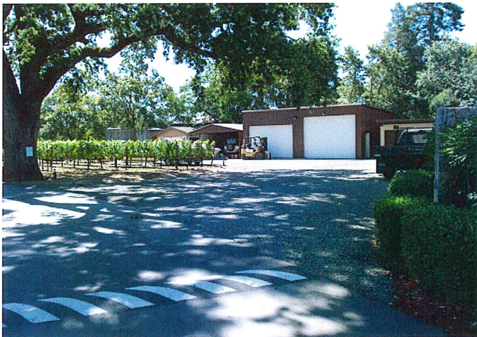
Photograph 26: Southeasterly panoramic view of existing structures. June 18, 2014
