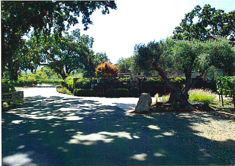
Photograph 19: Southeasterly panoramic view of existing driveway at residence. June 18, 2014
