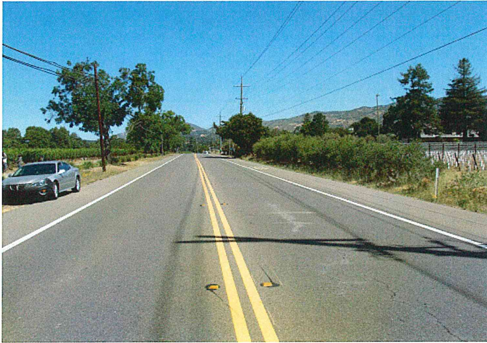
Photograph 17: Northerly view of Silverado Trail. June 18, 2014
