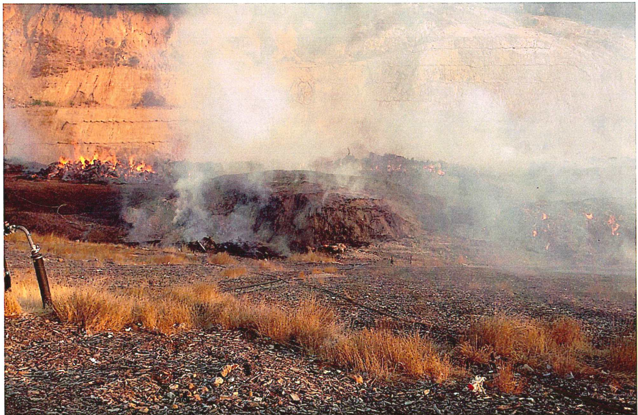
Ground green waste, wood waste & food waste Loss of piping on approx. 4 methane wells.
