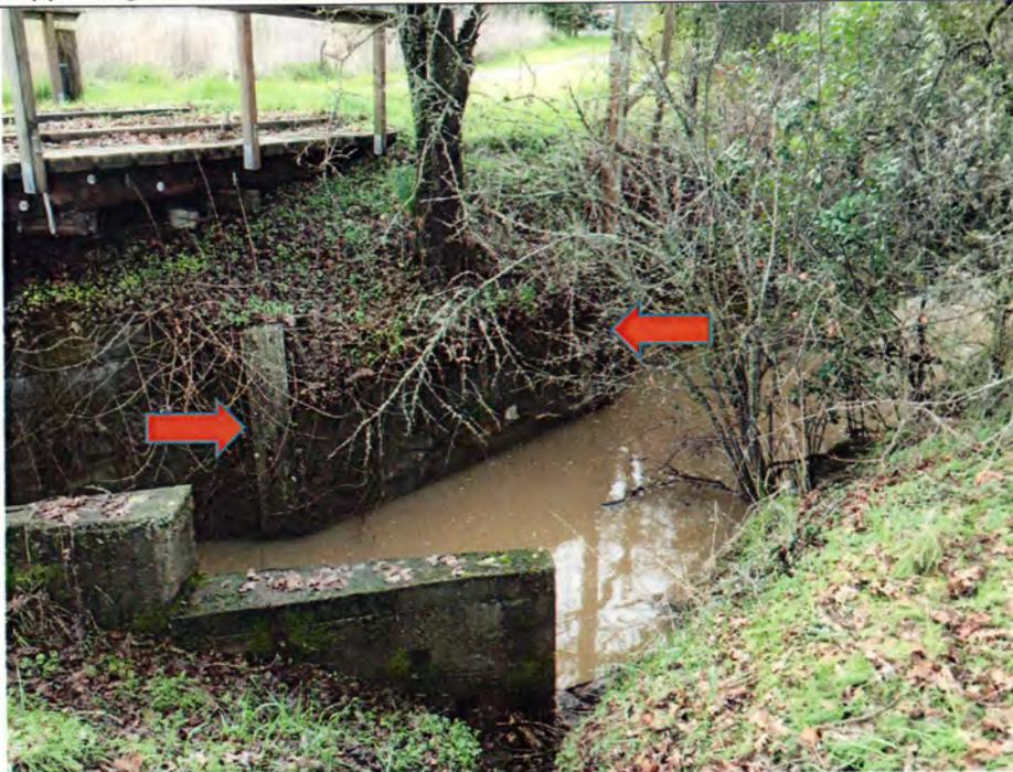
This 10 foot section of existing wall may remain, to provide necessary erosion scour protection. If it is deemed too weak to stand in place, it will be replaced with VRSS. Any replacement material will not exceed 1 cubic yard per running foot of stream. Avoidance of fill and in-stream construction activity will also void the need to acquire a Section 404 federal permit from USACOE.
