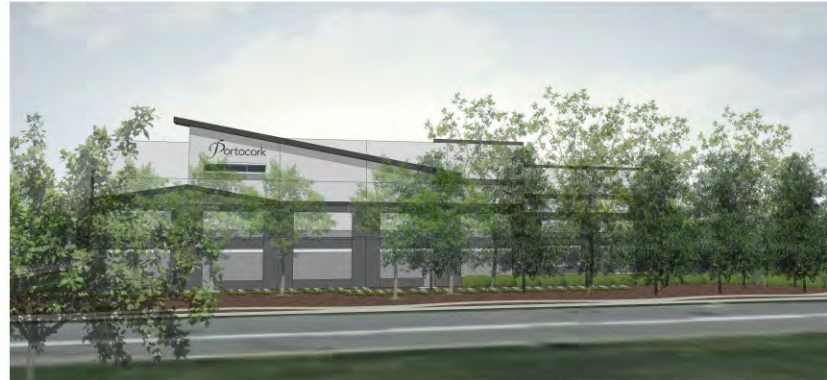
E. EAST BUILDING FACADE WITH LANDSCAPE SCREENING
