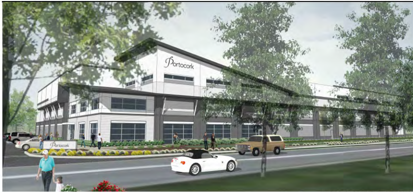
B. VIEW OF SOUTH BUILDING FACADE
