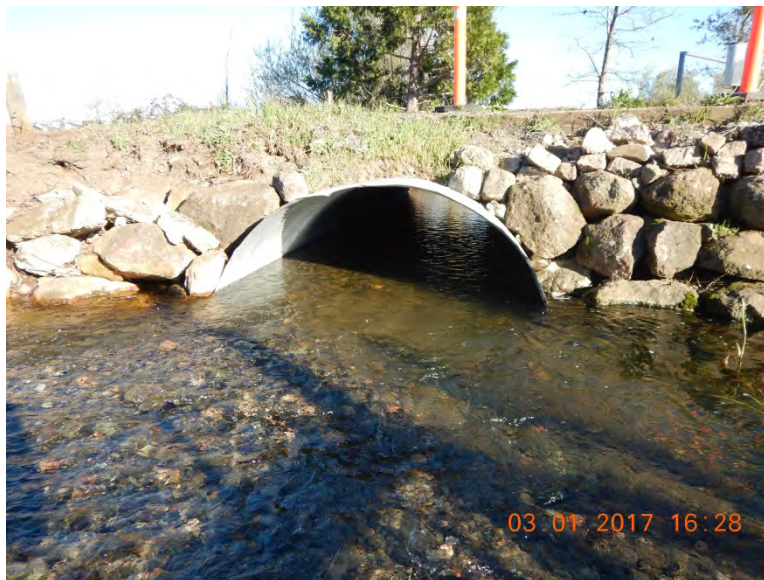
Photo 1: Bale Slough 72" CMP Culvert at South Whitehall Lane.
