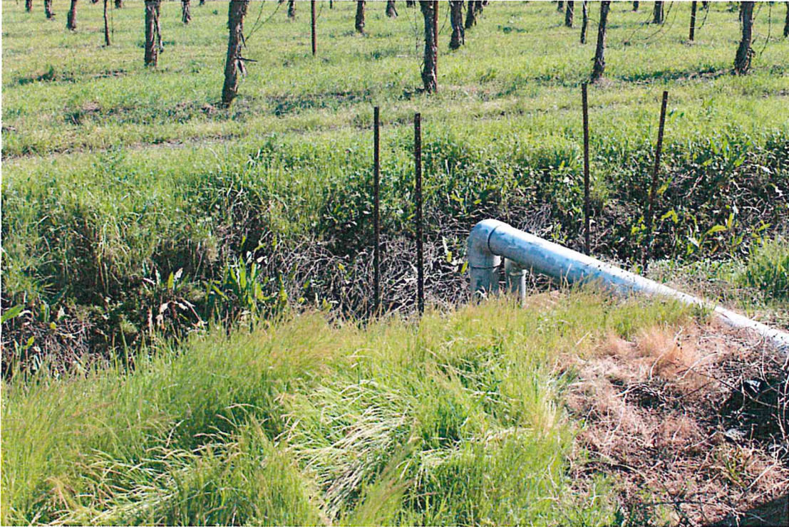
Photo 5: Drainage ditch northeast of Sullivan property.
