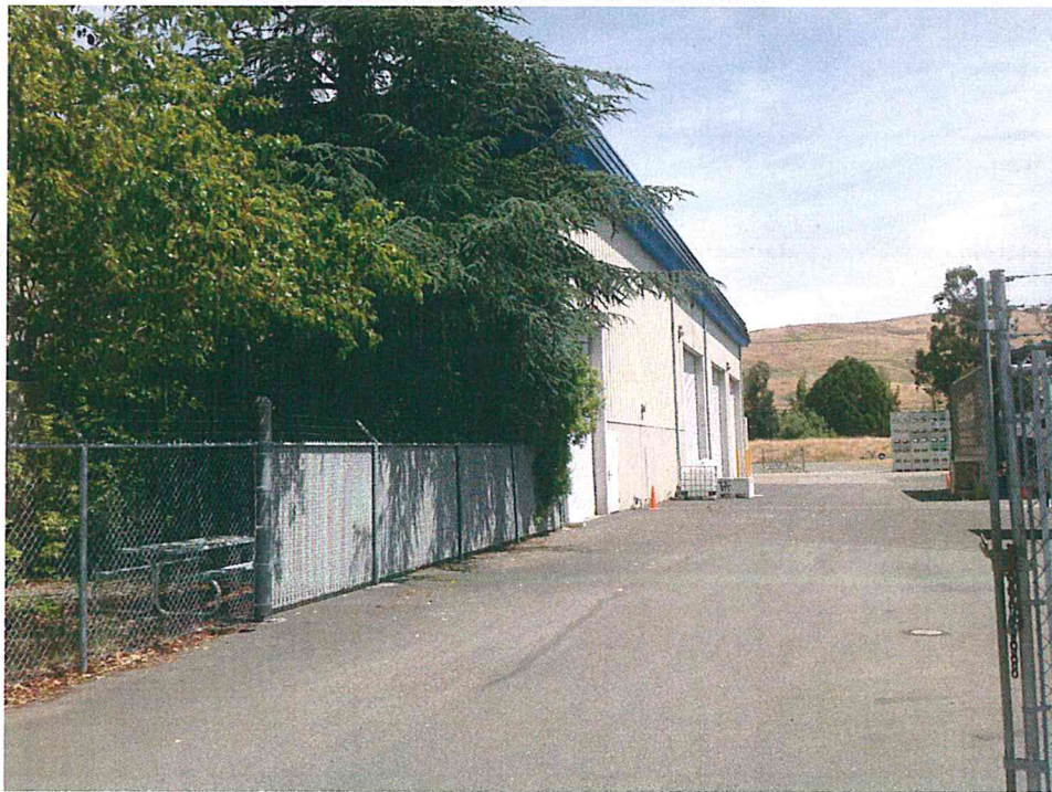
SOUTH SIDE OF BUILDING
