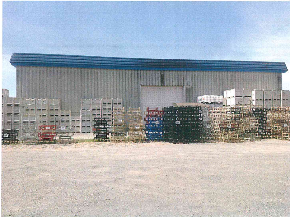
WEST SIDE OF BUILDING
