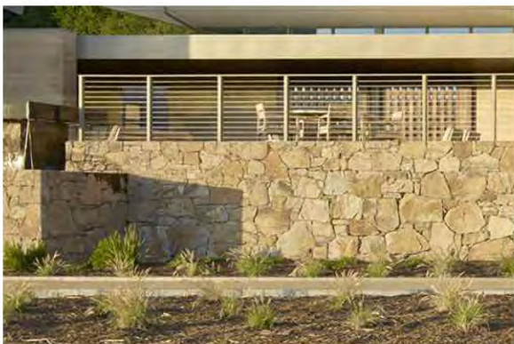
CUT STONE RETAINING WALLS & SEAT WALLS
