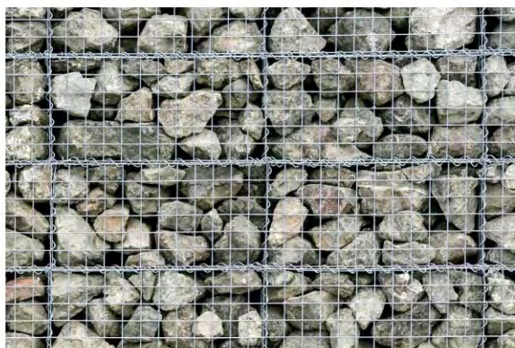
GABION RETAINING WALLS W/ ROCK FROM CAVE EXCAVATION
