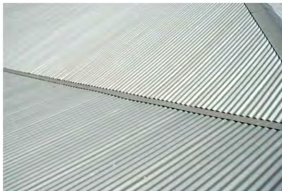
CORRUGATED METAL ROOFING
