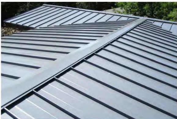
STANDING SEAM METAL ROOFING
