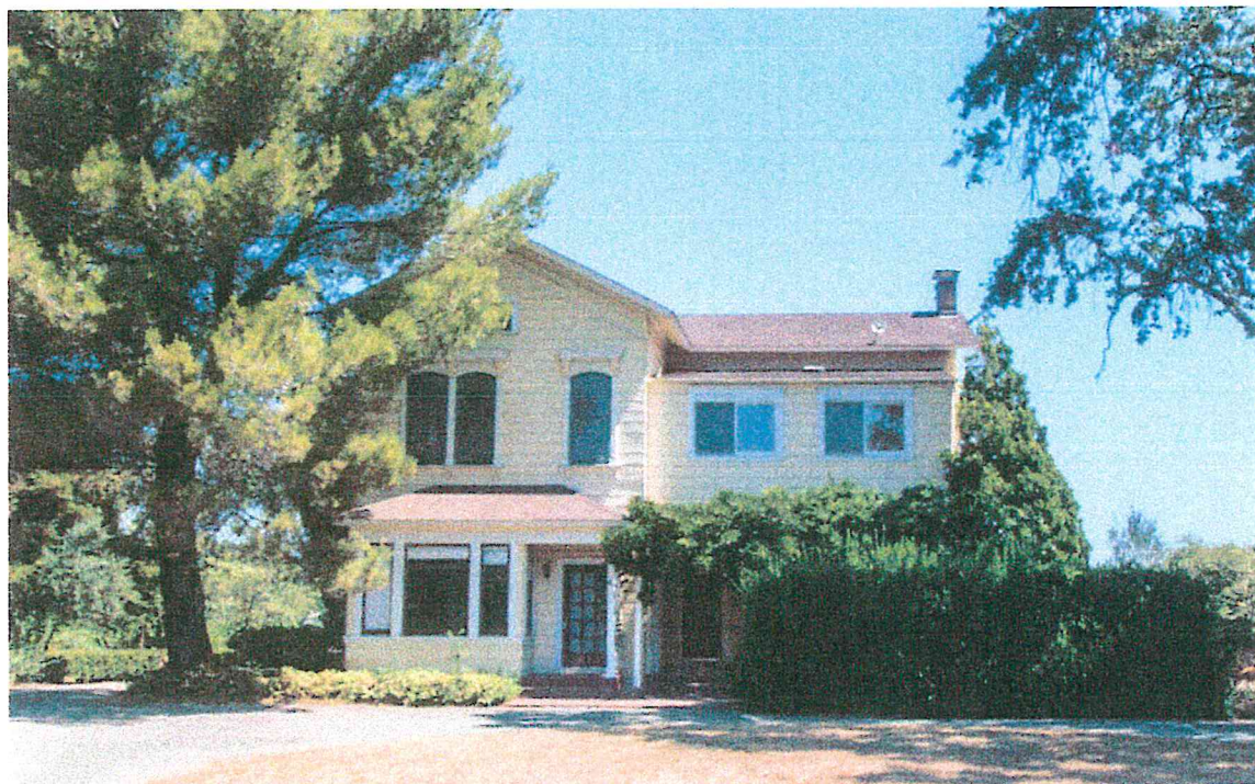
Main residence, west (primary) facade, detail (Architectural Resources Group, August 2015)
