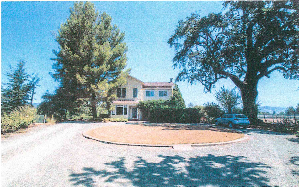
Main residence, west (primary) facade (Architectural Resources Group, August 2015)
