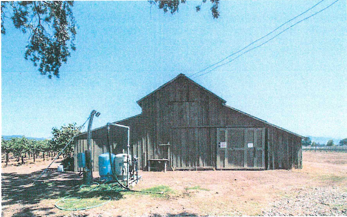
Barn, west facade (Architectural Resources Group, August 2015)
