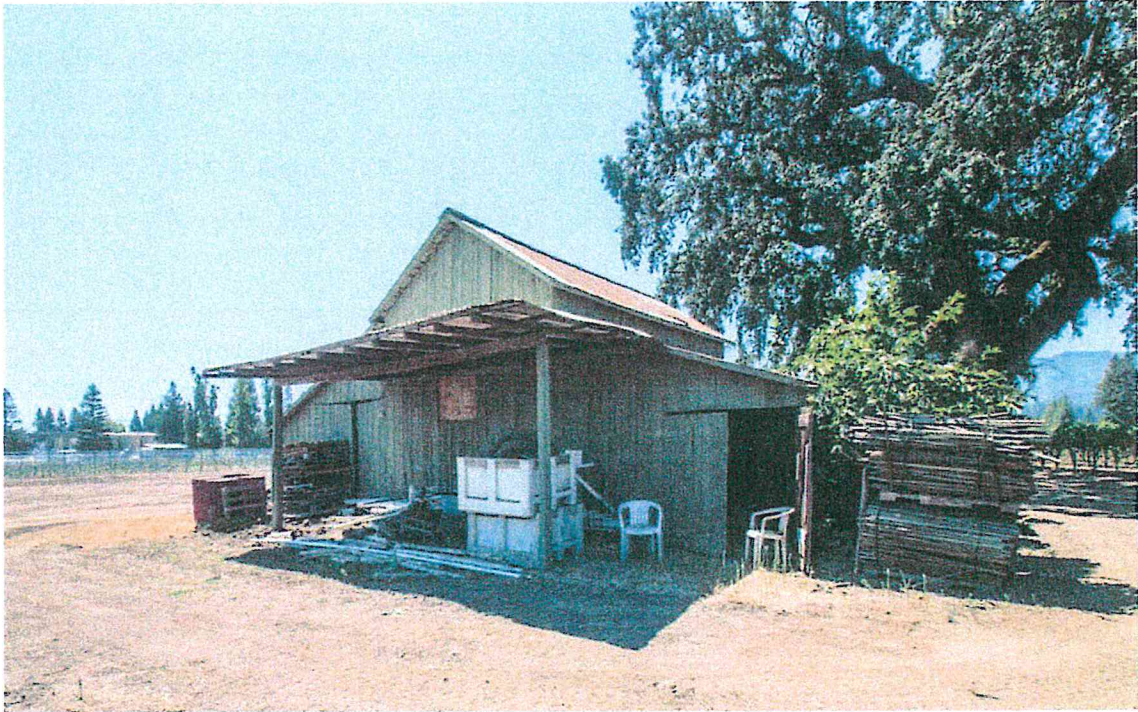
Barn, east facade (Architectural Resources Group, August 2015)
