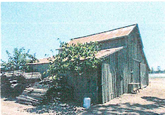
Figure 7. Barn, north and west façades (Architectural Resources Group, August 2015)
