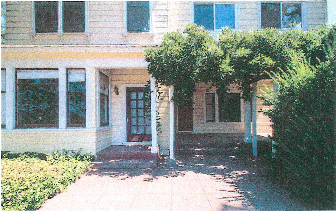
Main residence, west facade (Architectural Resources Group, February 2015)
