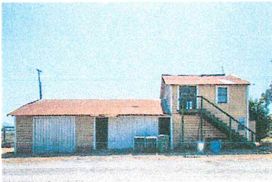
Figure 5. Guest House/Shed, north façade (Architectural Resources Group, August 2015)
