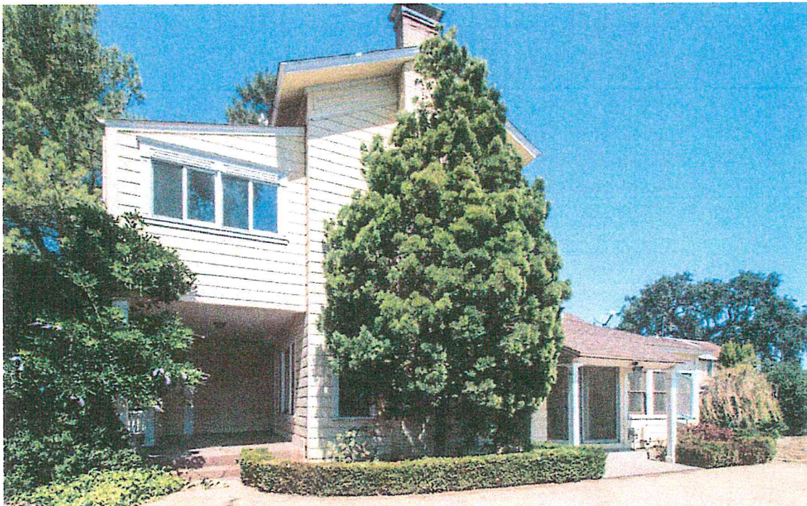
Main residence, south facade (Architectural Resources Group, August 2015)
