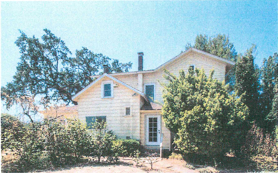
Main residence, east facade (Architectural Resources Group, August 2015)
