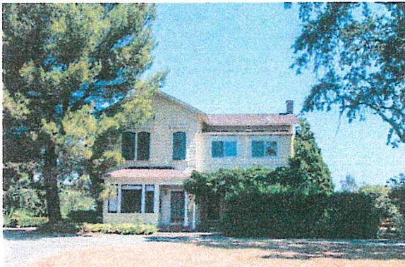
Figure 3. Main Residence, west façade (Architectural Resources Group, August 2015)
