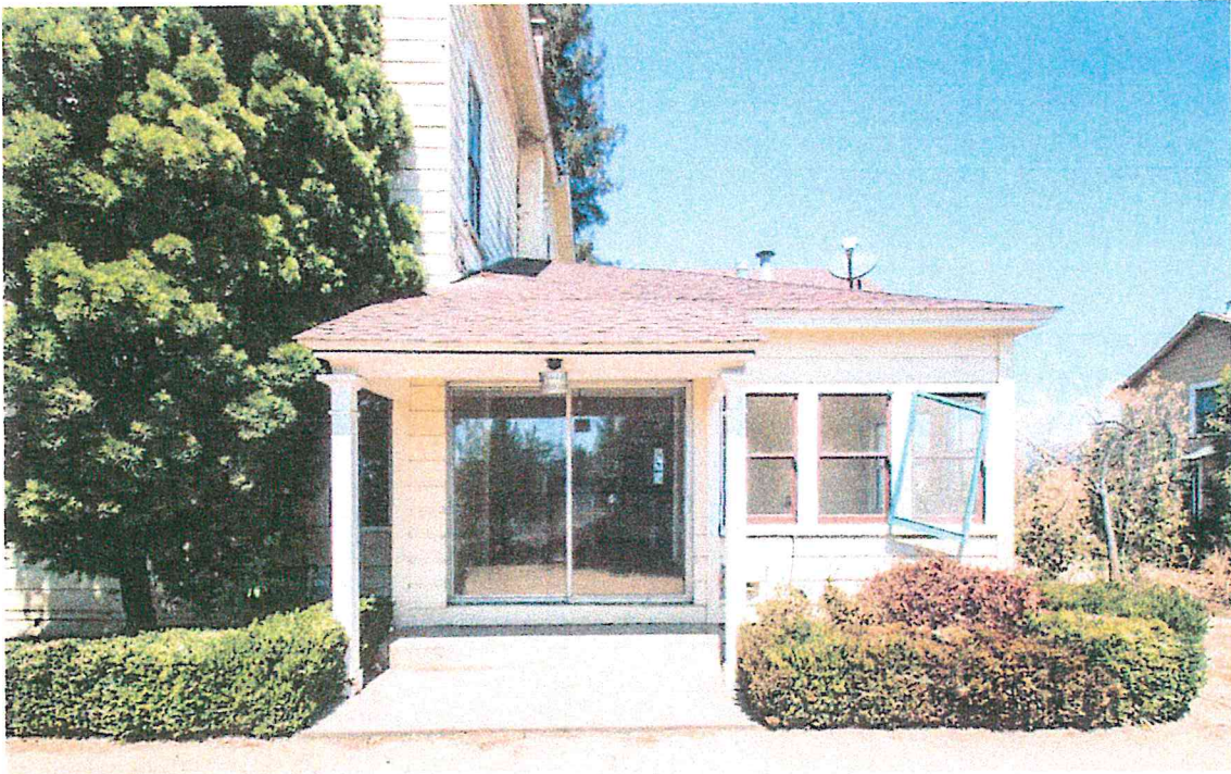
Main residence, south facade, detail (Architectural Resources Group, August 2015)
