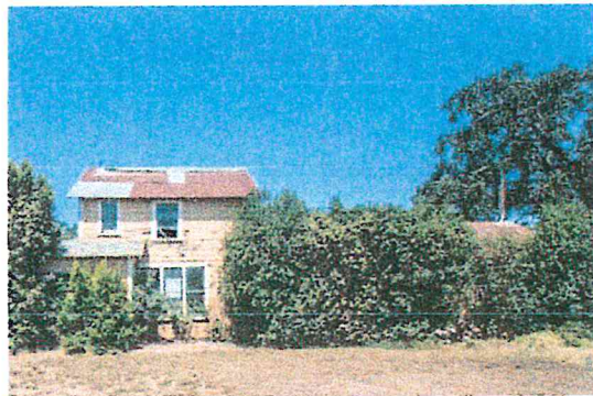
Figure 6. Guest House/Shed, south façade (Architectural Resources Group, August 2015)
