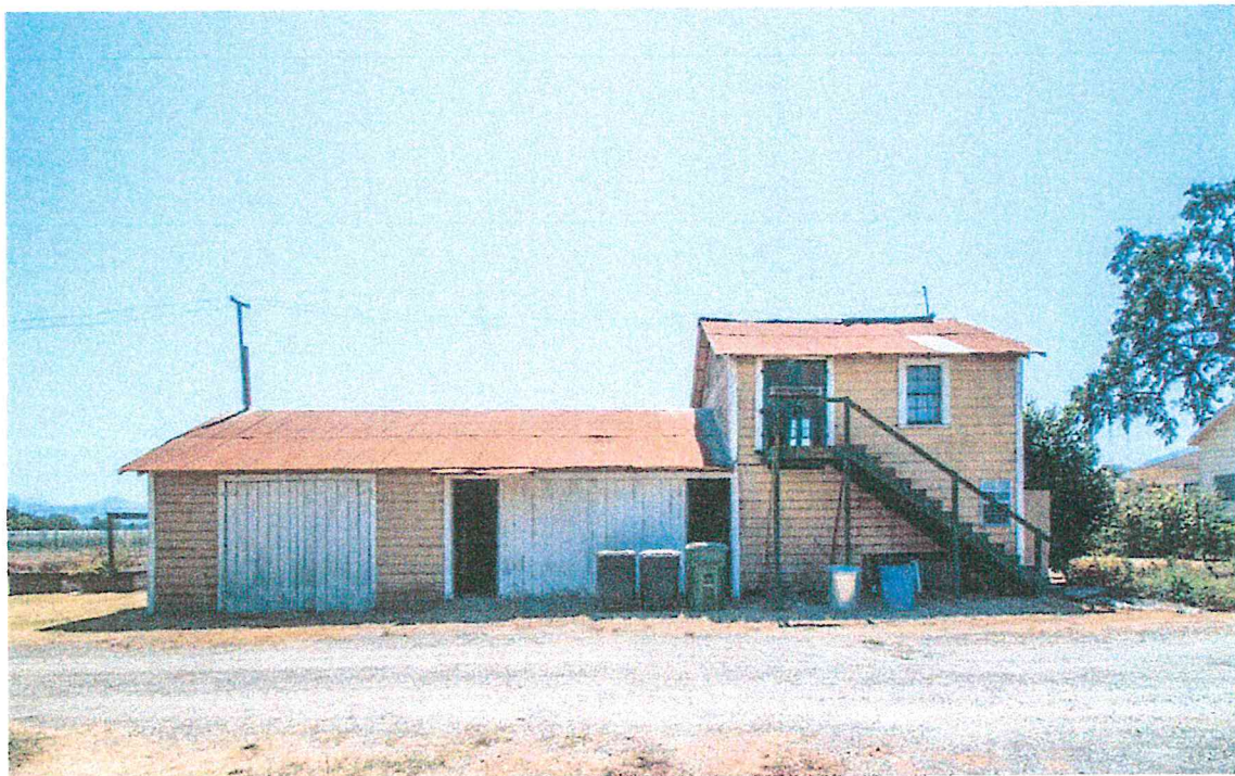
Guest house, north facade (Architectural Resources Group, August 2015)
