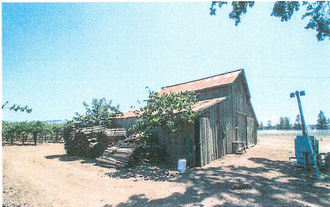
Barn, north and west facades (Architectural Resources Group, August 2015)
