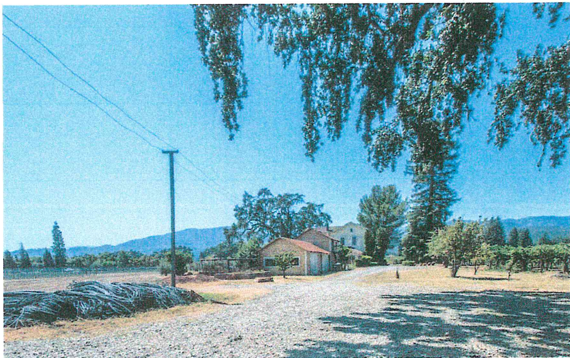
Guest house and main residence, view looking west from barn (Architectural Resources Group, August 2015)
