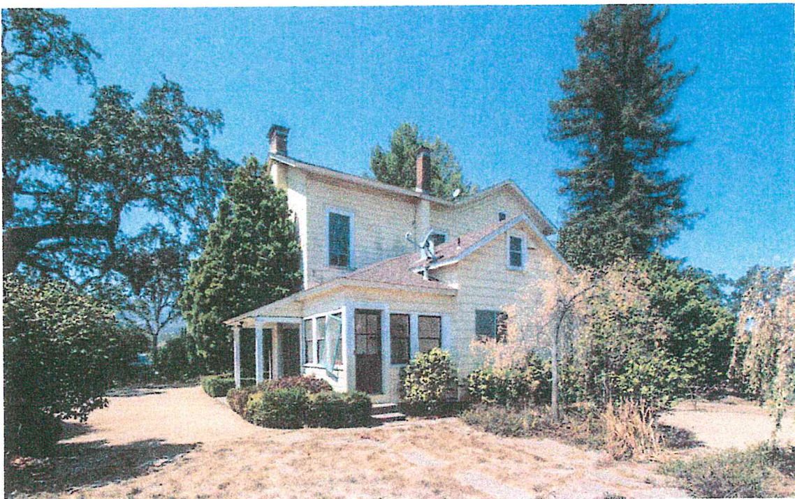
Main residence, south and east facades (Architectural Resources Group, August 2015)
