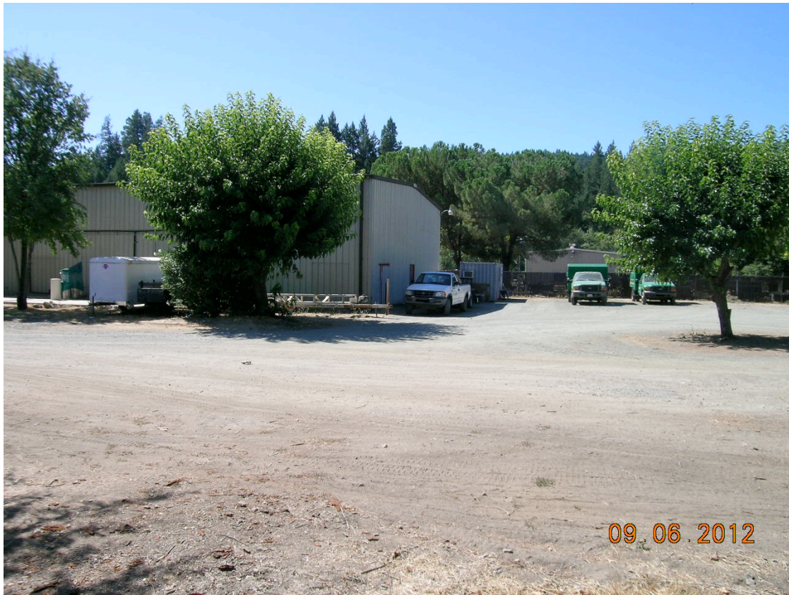
Figure 2. View of existing structures to be removed.
