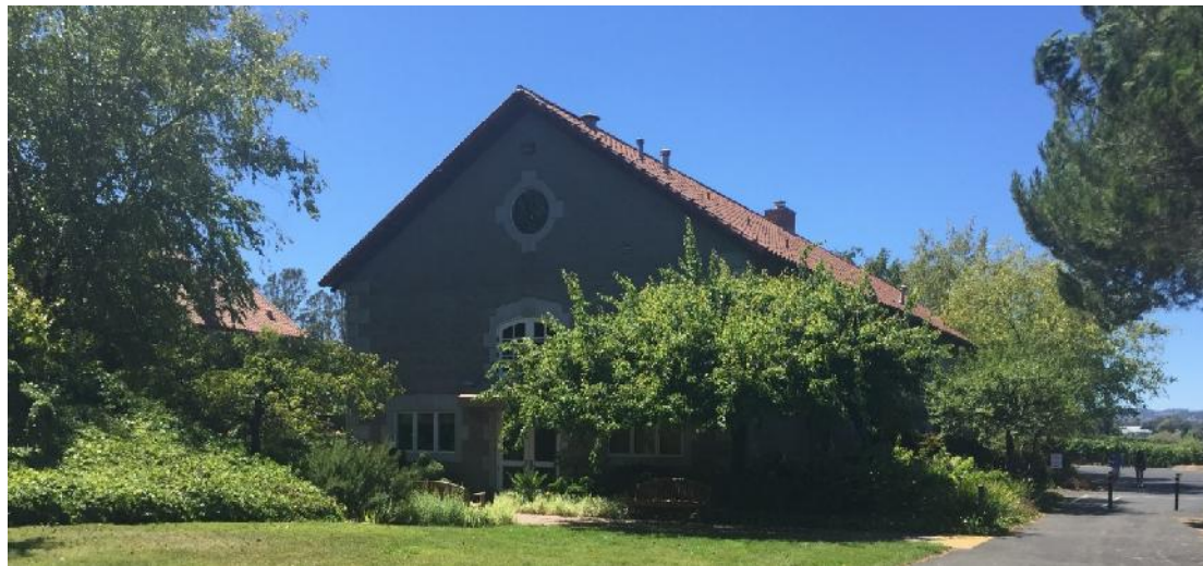
View of Hospitality Building from the South (8/12/2015)
