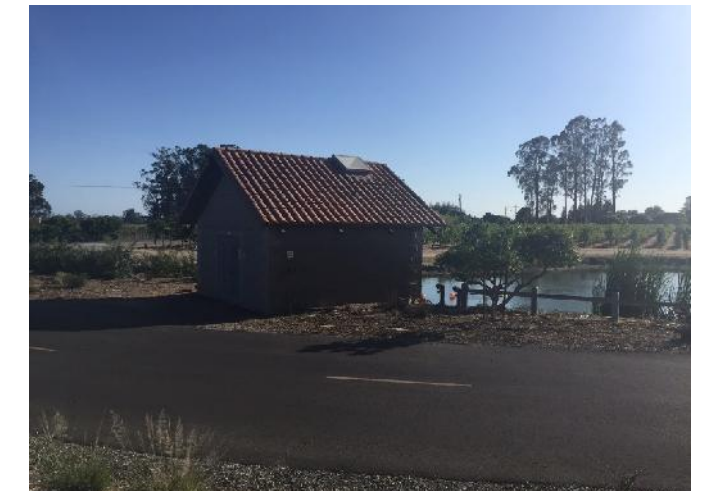
View of Fire Pump House from the East (9/3/2015)
