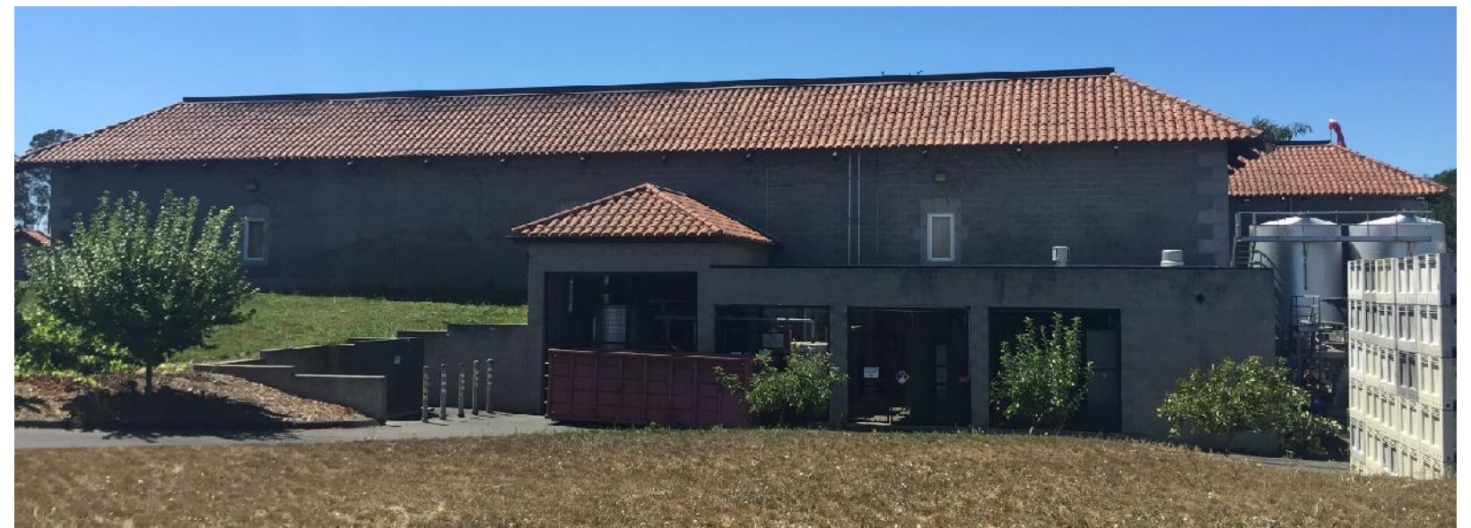
View of Main Production Building and Mechanical Room from the South (8/12/2015)
