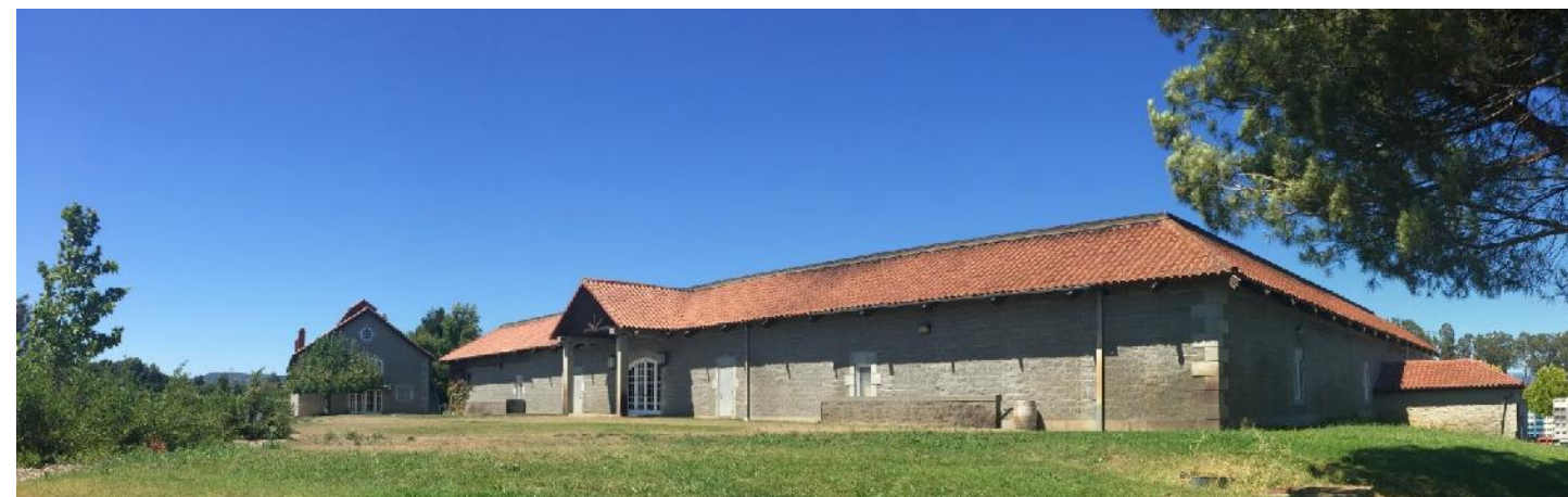
View of Main Production Building and Still House from the South West (8/12/15)
