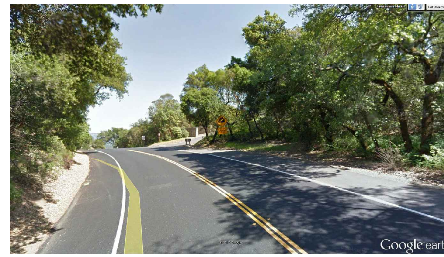
STA 2+00 (E) CONDITION - LOOKING EAST
