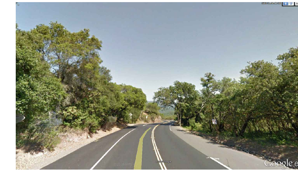
STA 5+00 (E) CONDITION - LOOKING EAST
