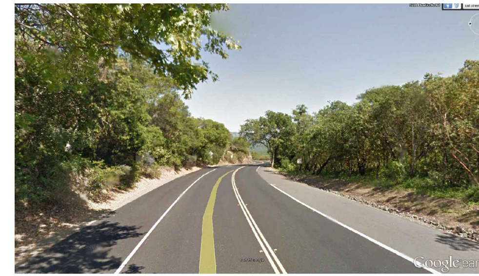
STA 4+50 (E) CONDITION - LOOKING EAST
