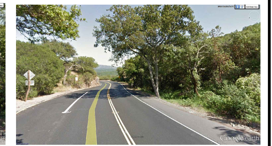
STA 6+00 (E) CONDITION - LOOKING EAST
