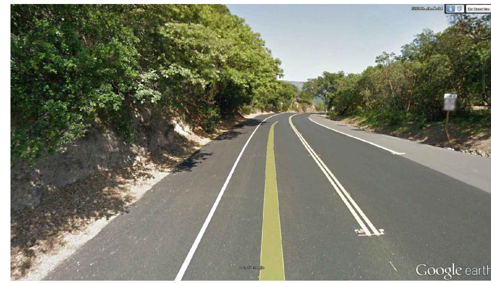
STA 3+50 (E) CONDITION - LOOKING EAST
