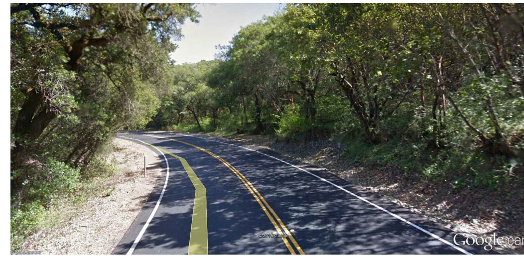
STA 0+00 (E) CONDITION - LOOKING EAST
