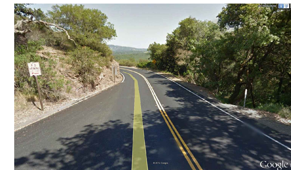
STA 7+00 (E) CONDITION - LOOKING EAST
