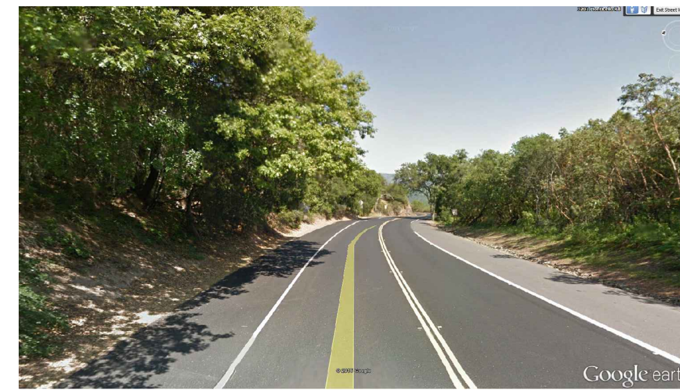
STA 4+00 (E) CONDITION - LOOKING EAST
