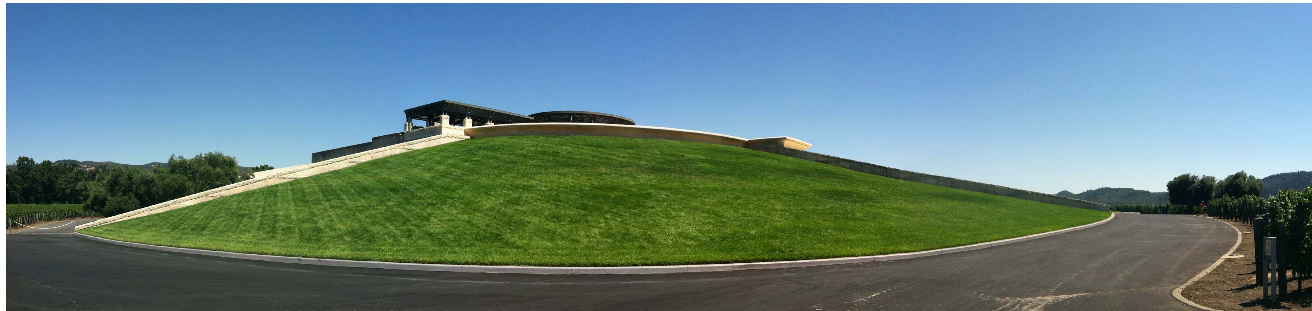
VIEW FROM SOUTHWEST DRIVEWAY
