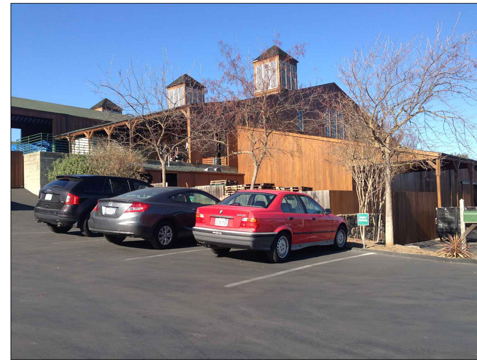
(F) VIEW OF THE PRODUCTION BUILDING FROM THE SOUTHEAST
