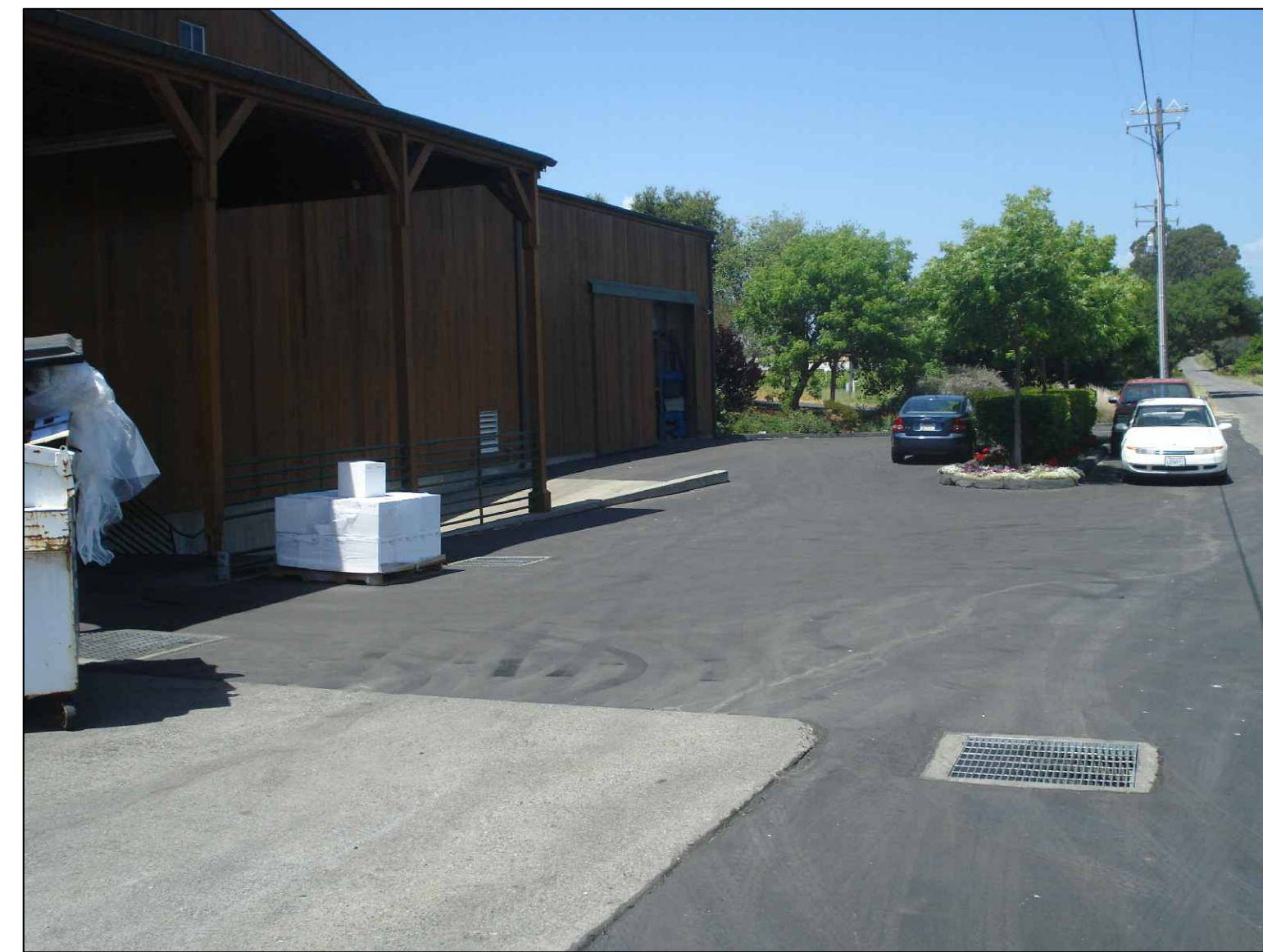
(H) VIEW OF THE PRODUCTION BUILDING LOADING DOCK FROM THE SOUTHEAST
