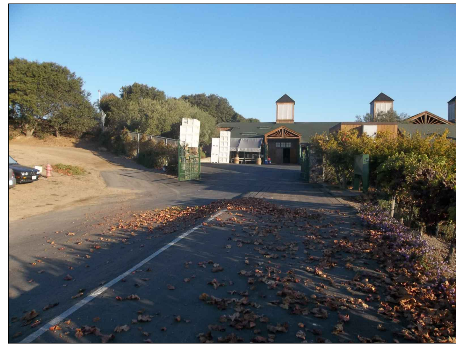
(B) VIEW OF THE PRODUCTION BUILDING FROM THE SOUTH
