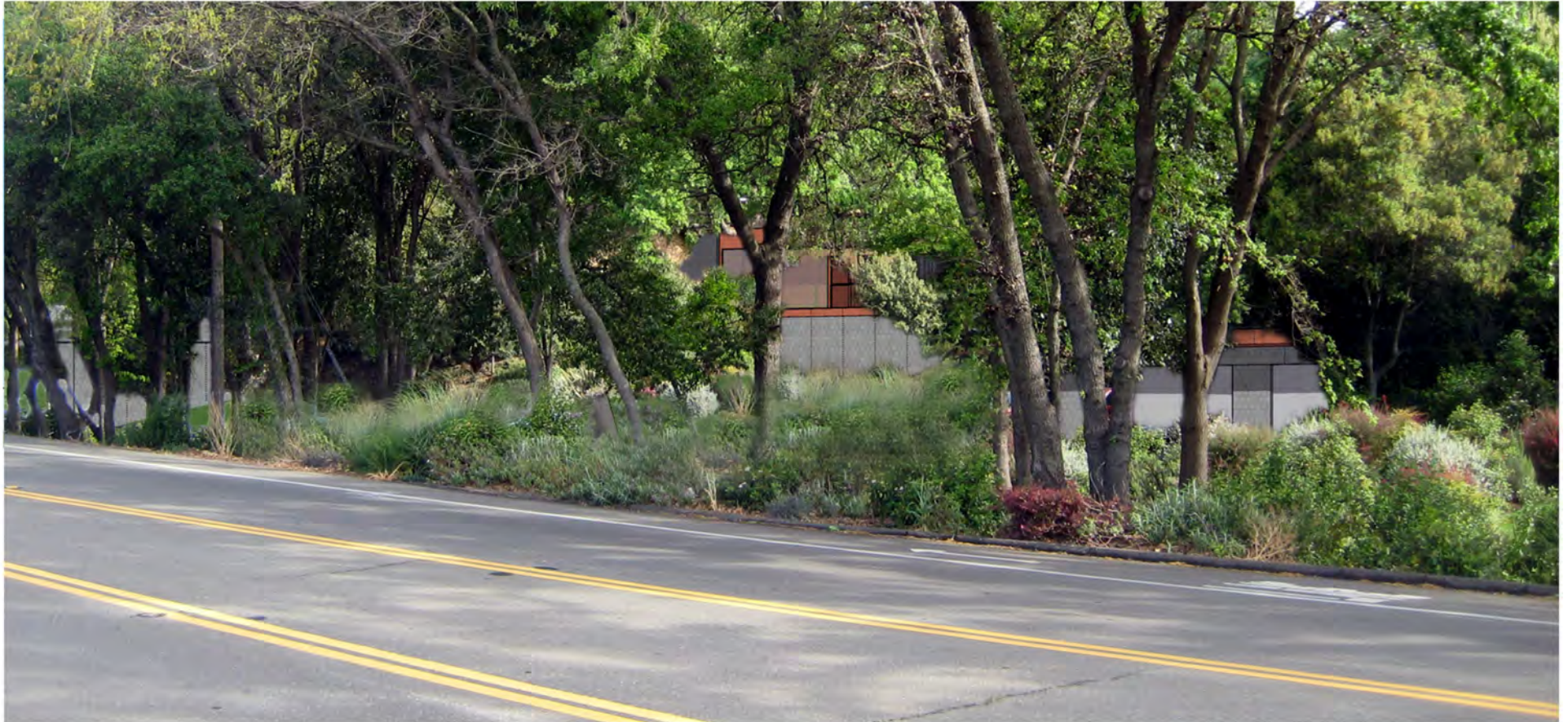
New Production Building from Silverado Trail
