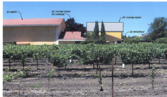
6 EXISTING WINERY - VIEW FROM TUBBS LANE NOT TO SCALE
