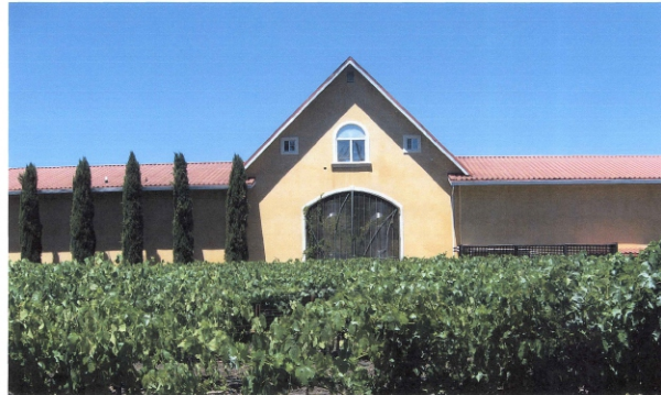
5 EXISTING WINERY - VIEW FROM TUBBS LANE NOT TO SCALE
