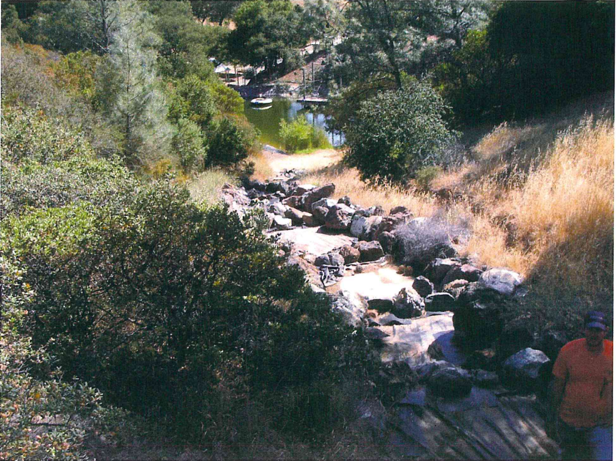
Photograph 1: Rocks situated in straight lines to form pools. Upon removal of the plastic lining, these rocks would be slightly modified to reflect a more natural streambed condition.
