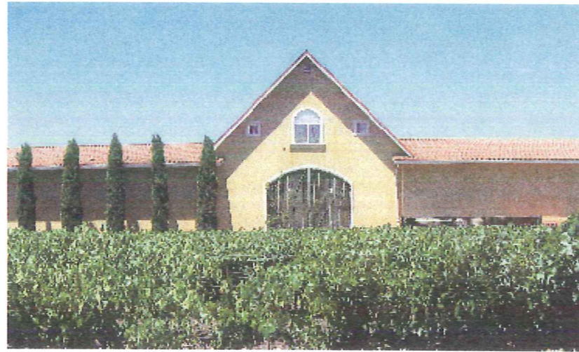
5 EXISTING WINERY - VIEW FROM TUBBS LANE SCALE 1/8" = 1'-0"
