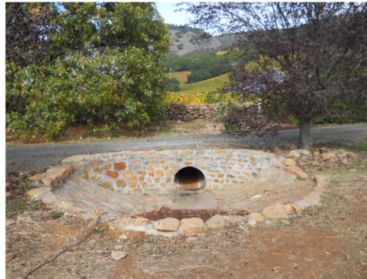
EXISTING DRAINAGE ALONG DRIVEWAY
