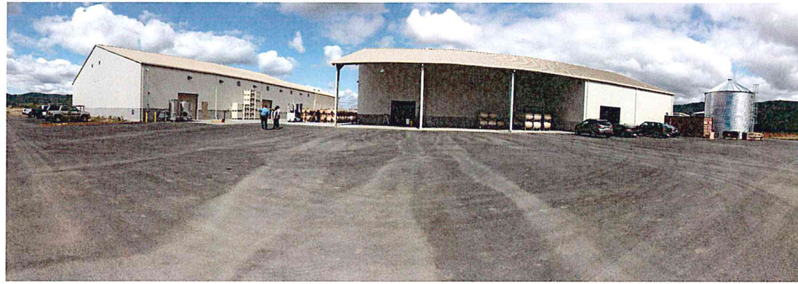
Winery, view of south side
