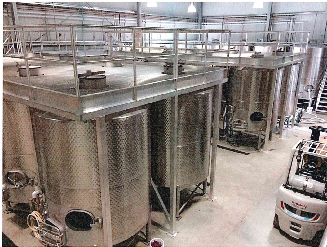
Winery Interior, Tank Storage
