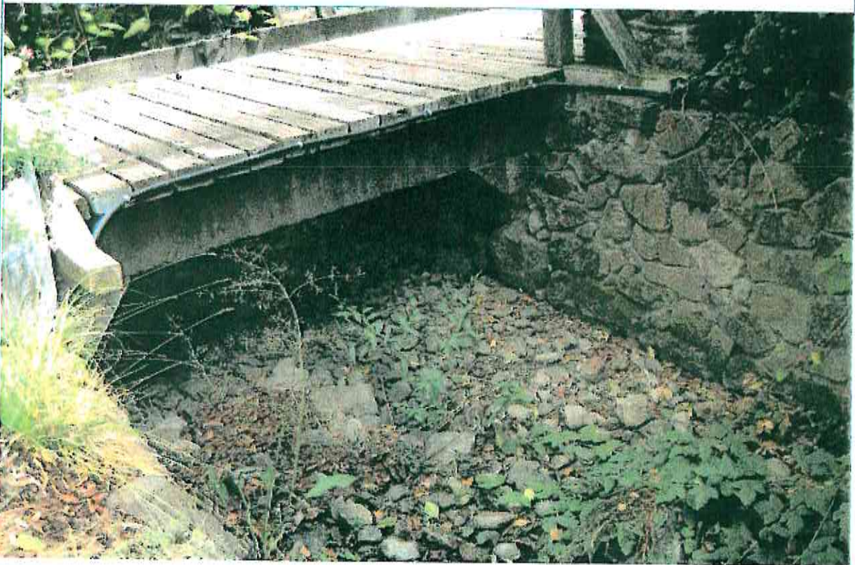
Photograph 20: Teal Creek footbridge
