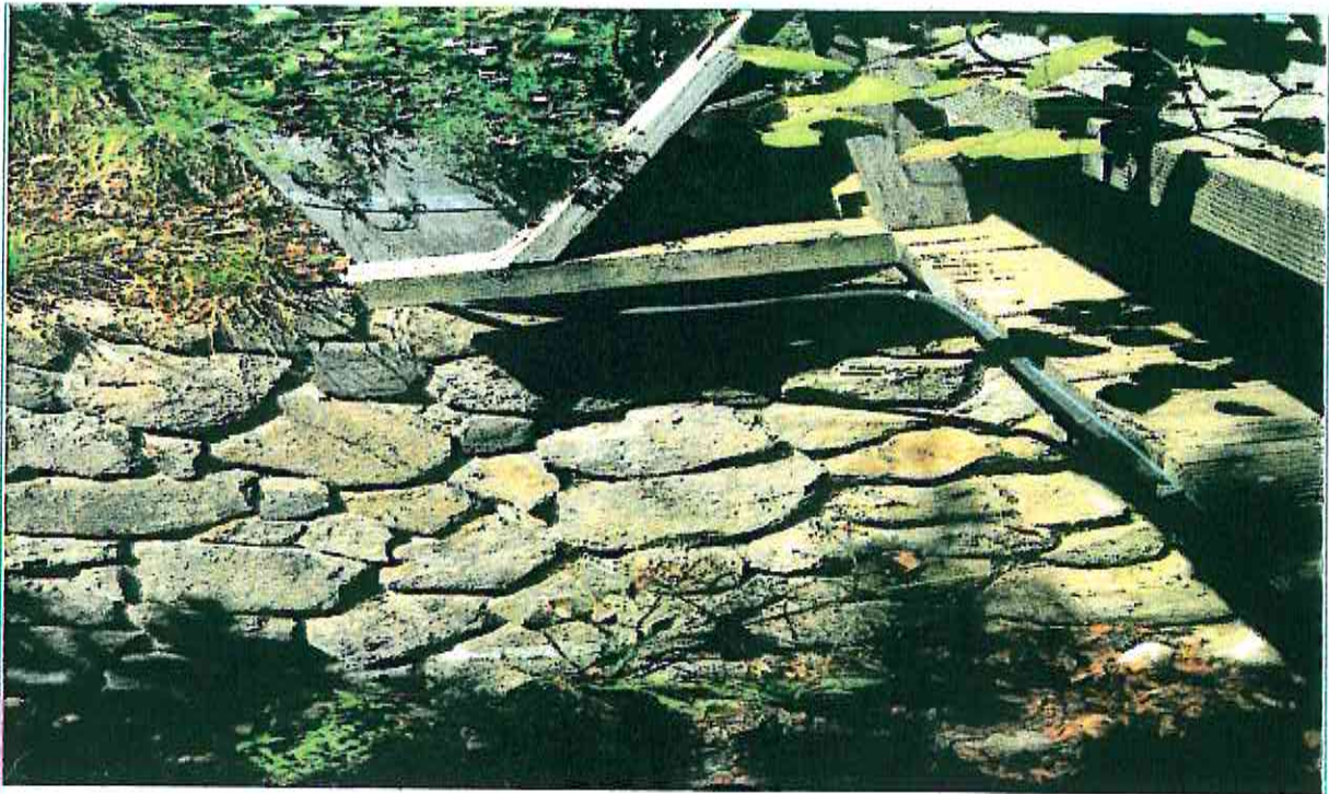
Photograph 11: Teal Creek footbridge
