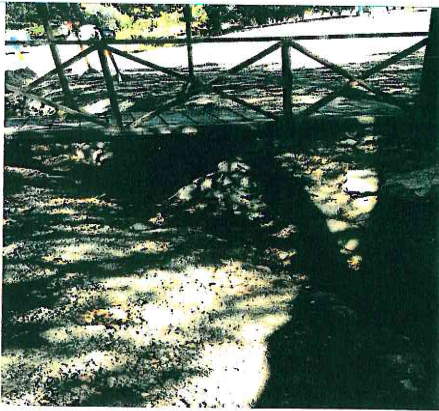
Photograph 1: Footbridge across unnamed drainage
