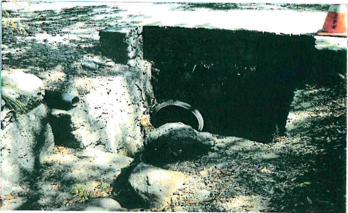
Photograph 3: Unnamed drainage illustrating culverts
