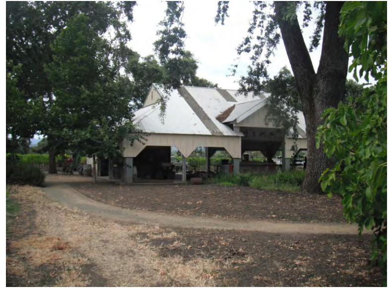
Looking Northeast at Pavilion
