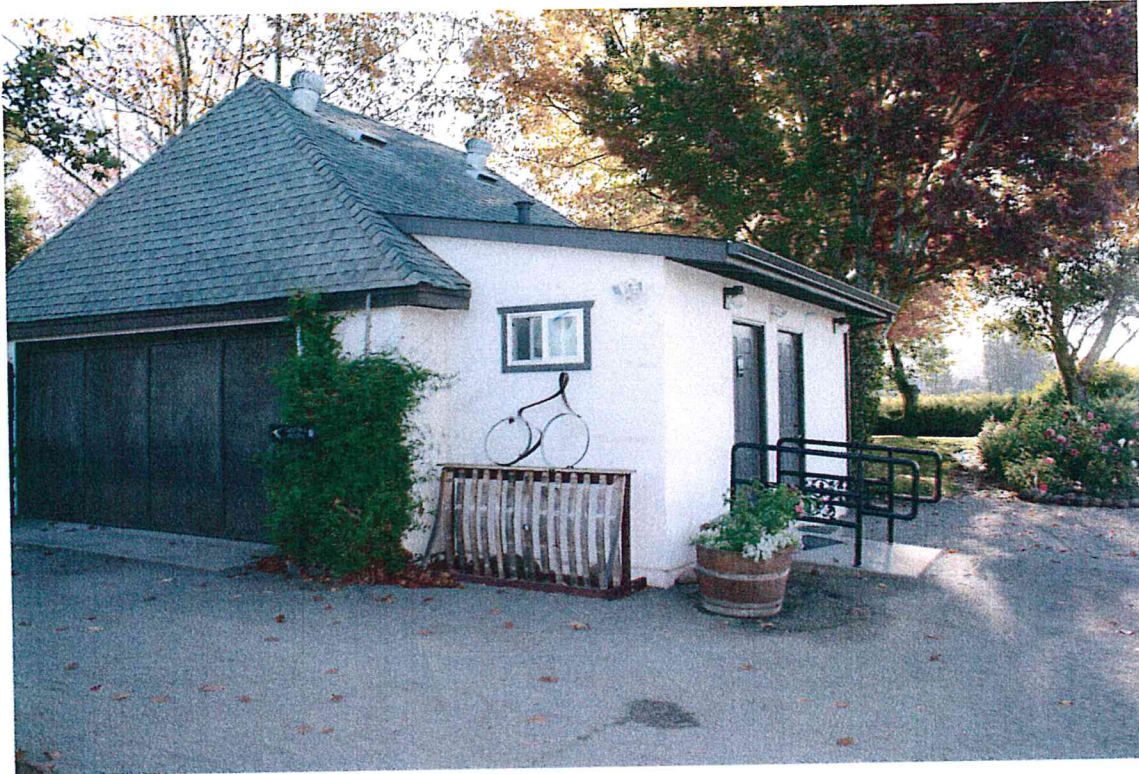
Existing house garage to be demolished
