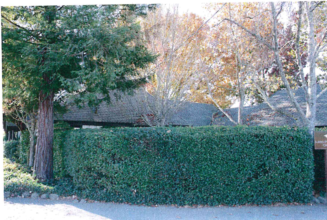
Existing house to be demolished
