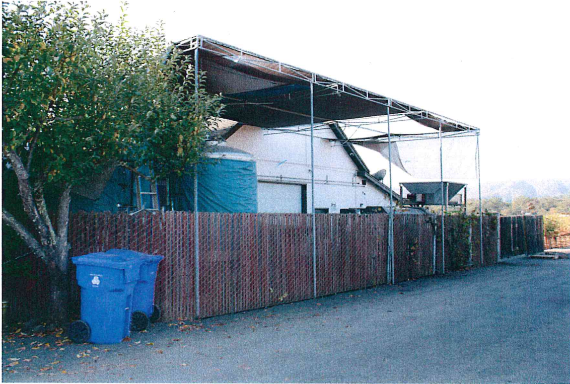
Existing winery tanks and crush area to be demolished
