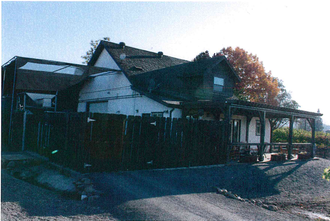
Existing winery to be demolished
