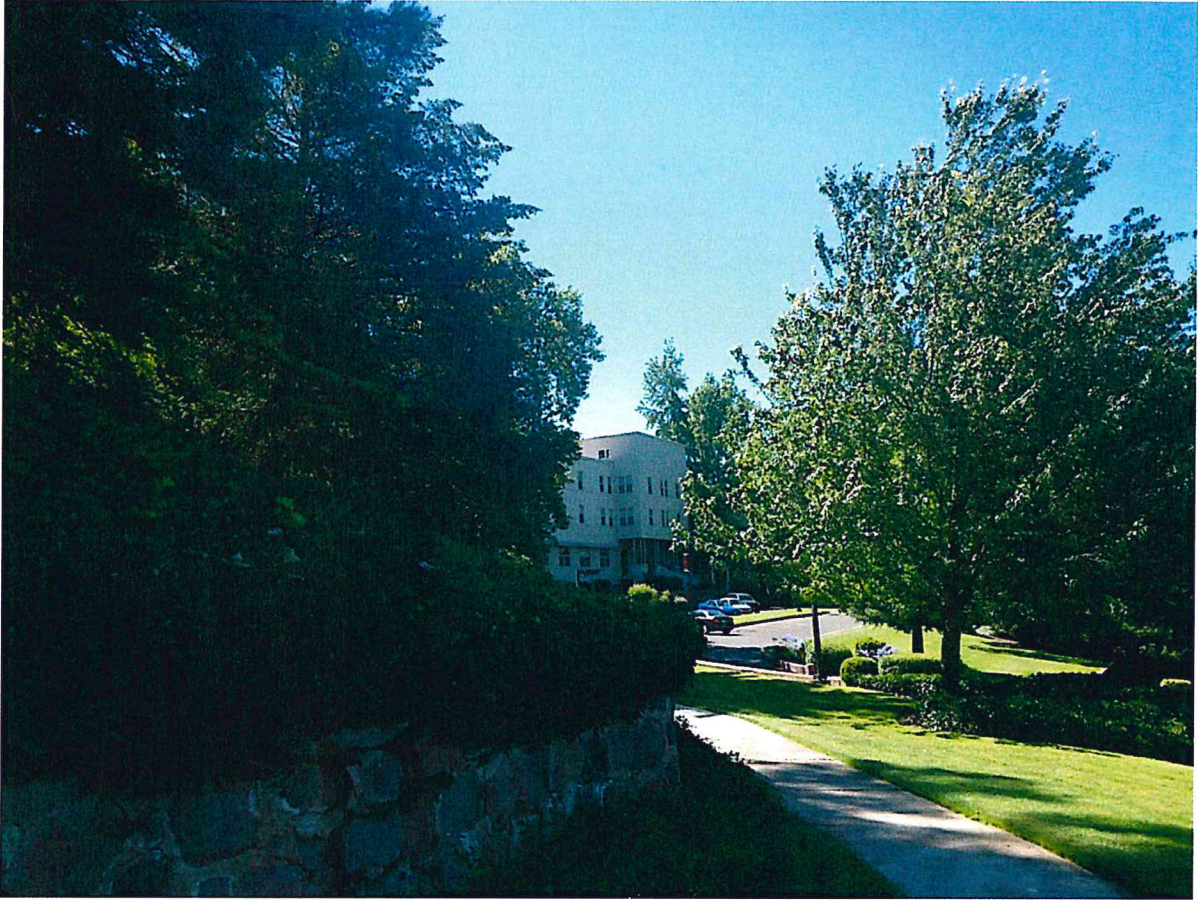
View west at building and parapet
