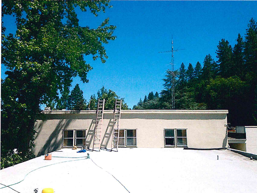
View north at penthouse, antennas go above, equipment inside
