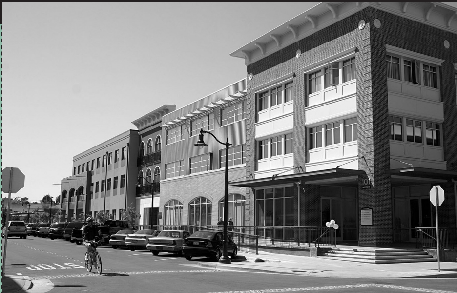
▼ Revitalizing Petaluma's downtown: Code for street front types (below), the new Boulevard Cinema (bottom left) and new mixed-use development (left).
