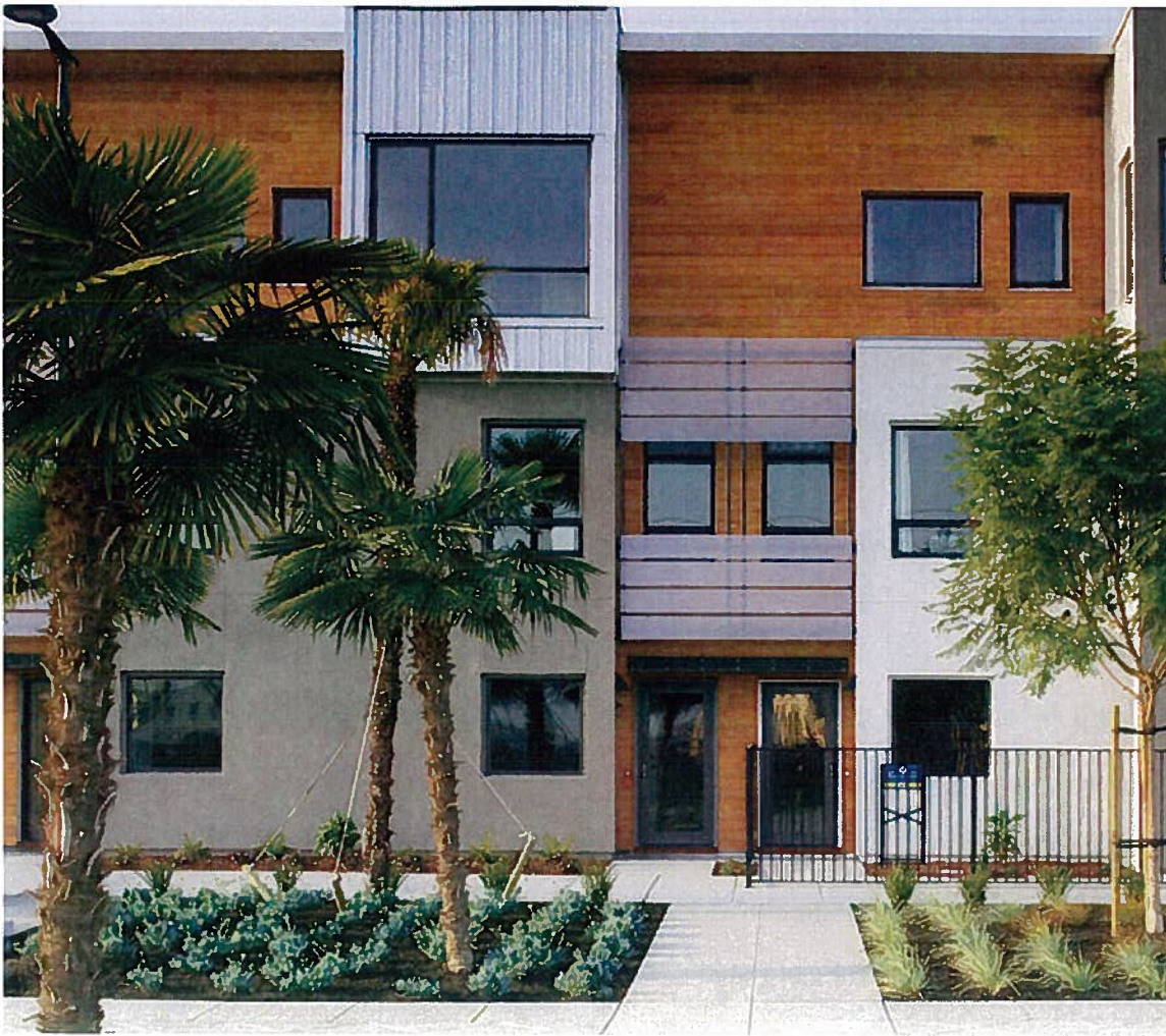
Townhouse entries facing interior courtyard
