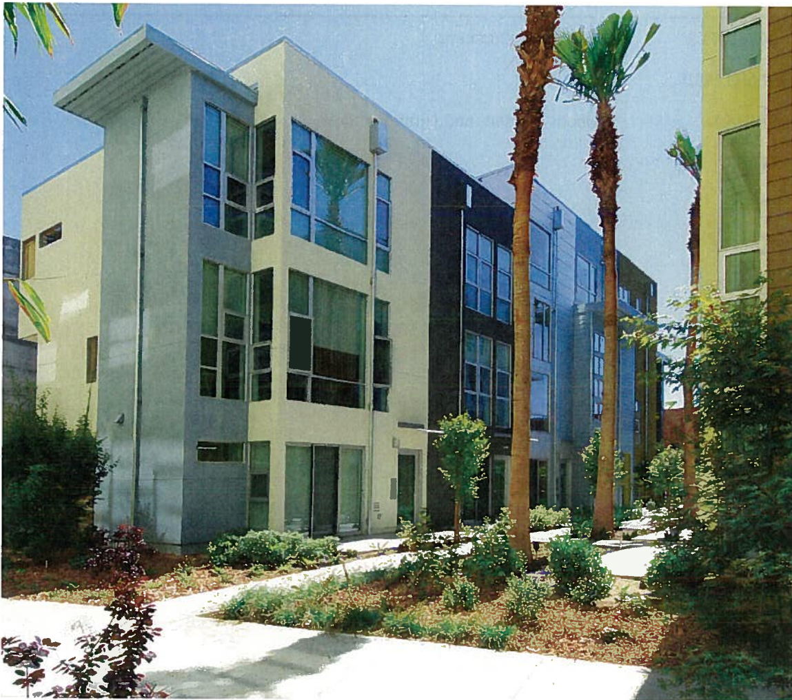
Townhouses facing interior mews
