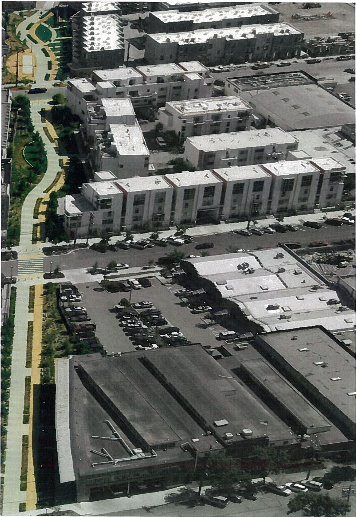
NAPA PIPE—SIMILAR PROJECTS TOUR | SITELAB urban studio
