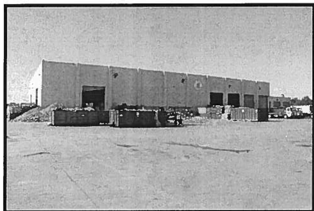
Collection Vehicle Access Doors on Left
