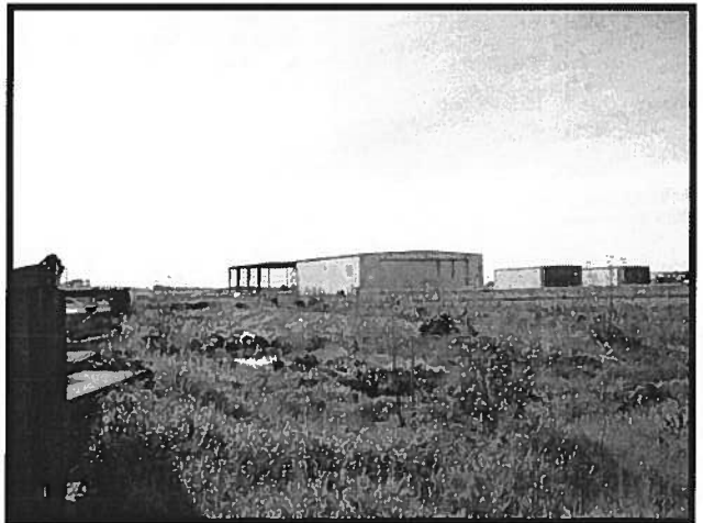
Figure 24. Partial View of Biofiltration Pond
