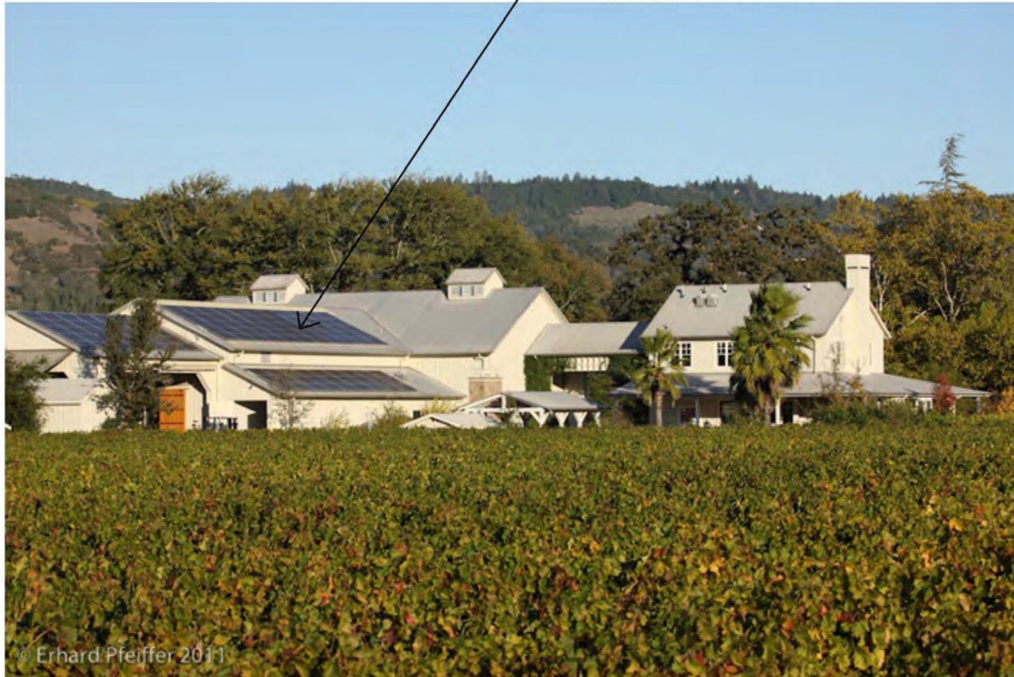
VIEW OF EXISTING WINERY FROM VINEYARD TO THE WEST
