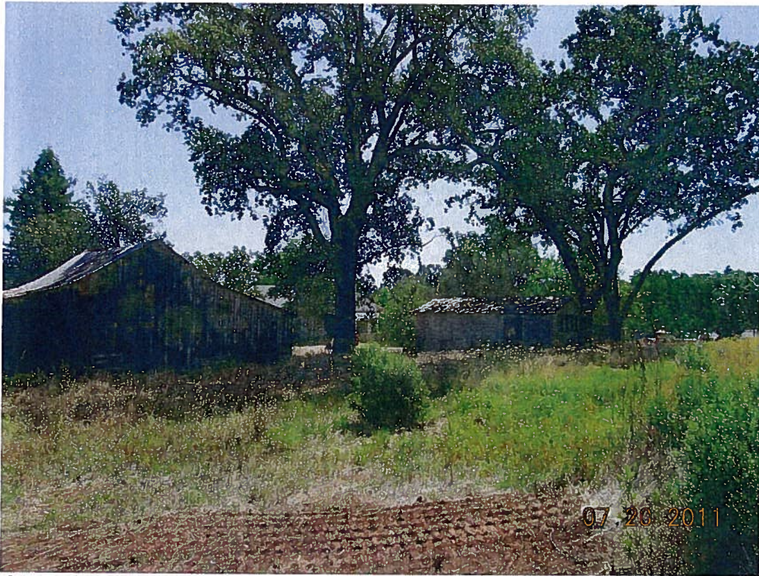
Figure 2. View of existing structures to be removed.
