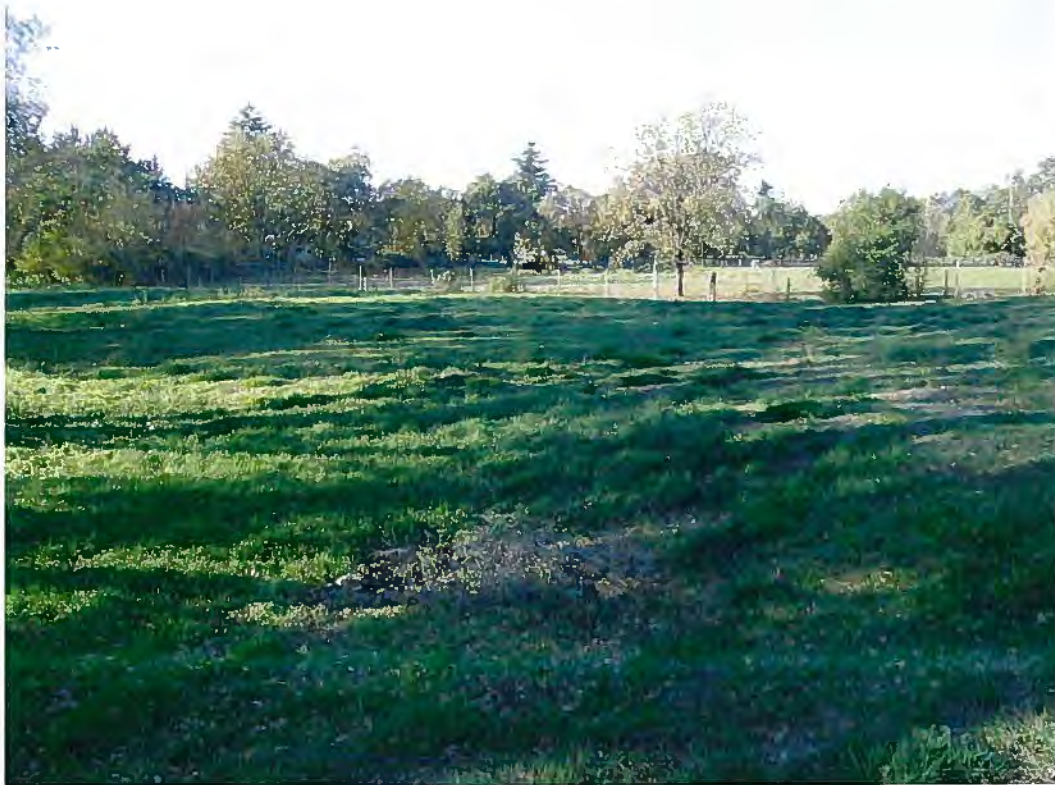
Photo 7. Location of storm-water retention, bio swale.
