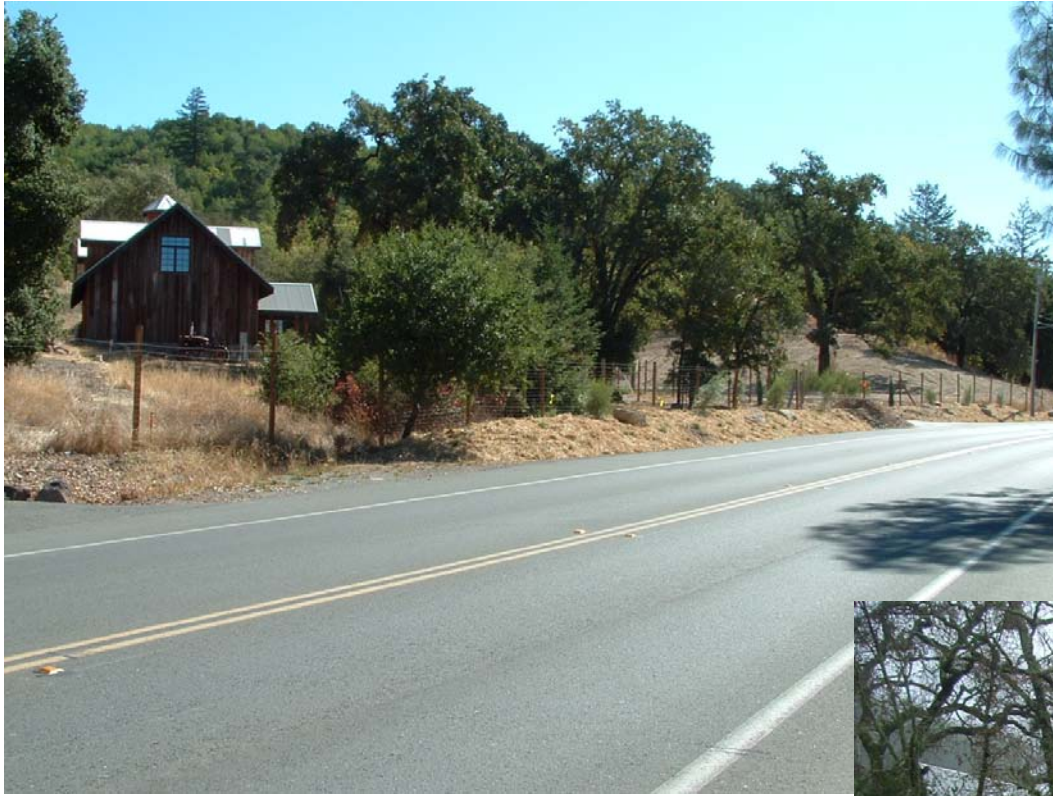
Silverado Trail Looking South Existing Ag Bldg.
