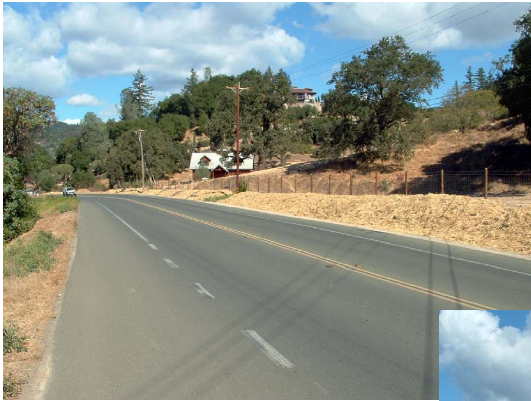
Silverado Trail Looking North Existing Ag Bldg
