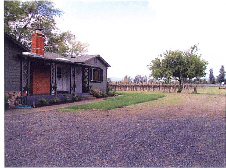
Photograph 19: Northwesterly panoramic view of existing residence, May 5, 2010
