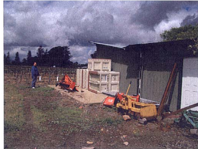
Photograph 3: Northerly panoramic view of existing barn, May 5, 2010
