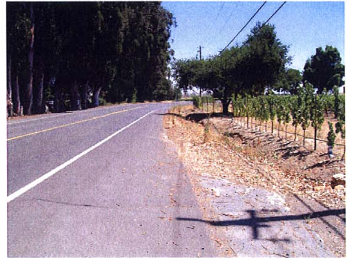
Photograph 27: Southeasterly view of existing driveway and Cuttings Wharf Road, July 19, 2010
