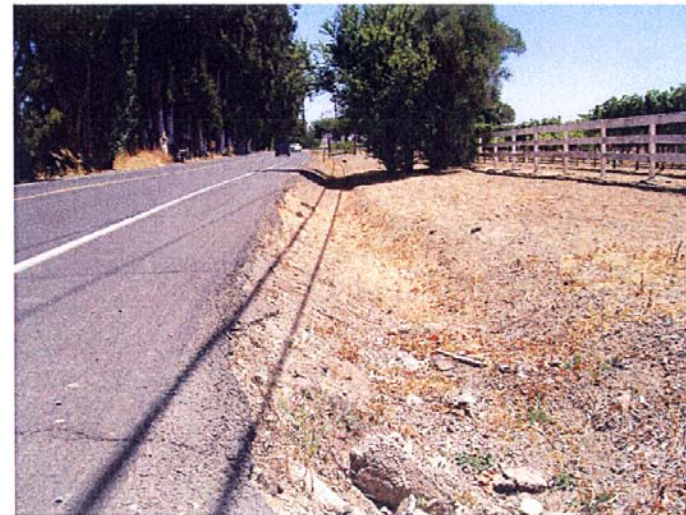
Photograph 31: Southeasterly view of Cuttings Wharf Road and existing drainage swale, July 19, 2010
