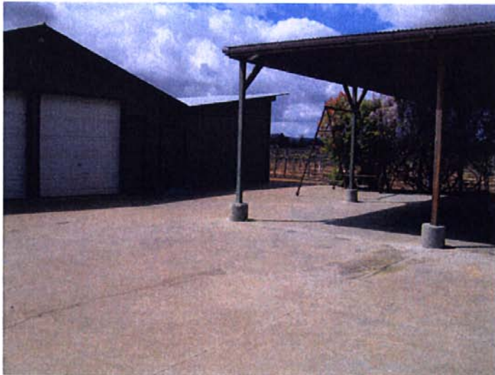
Photograph 6: Westerly panoramic view of existing barn and existing carport, May 5, 2010
