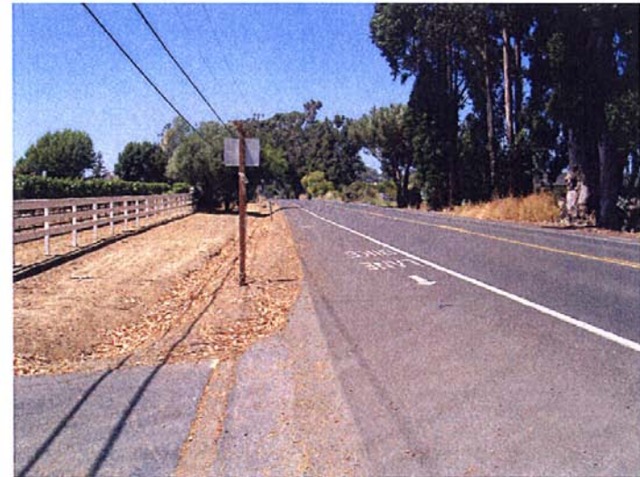
Photograph 28: Northwesterly view of existing driveway and Cuttings Wharf Road, July 19, 2010
