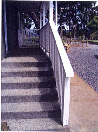
Photograph 17: Northeasterly panoramic view of existing southerly access to residence, May 5, 2010
