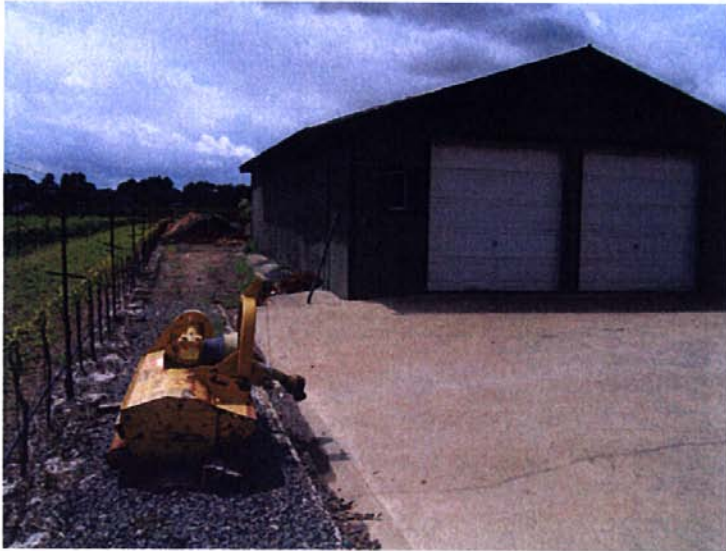
Photograph 5: Southwesterly panoramic view of existing barn May 5, 2010
