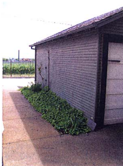
Photograph 14: Southerly panoramic view of existing storage building, May 5, 2010
