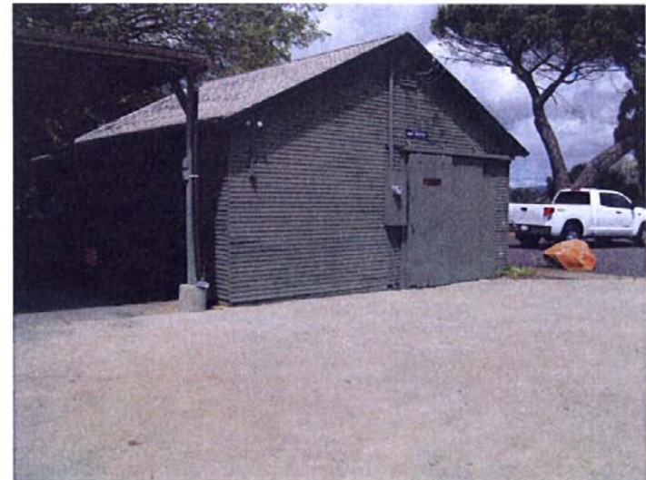
Photograph 8: Northerly panoramic view of existing carport and existing storage building, May 5, 2010
