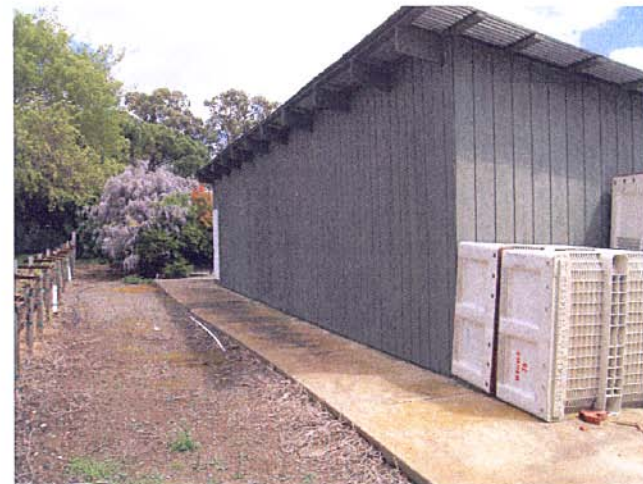
Photograph 4: Easterly view of existing barn, May 5, 2010
