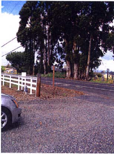
Photograph 25: Northerly panoramic view of existing driveway entrance at Cuttings Wharf Road, May 5, 2010
