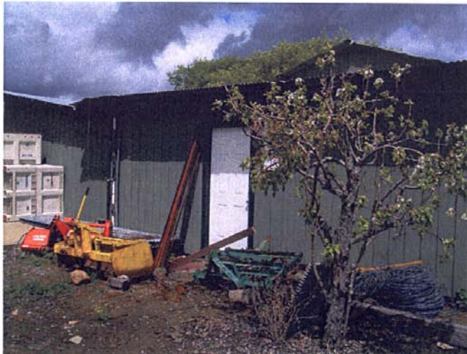
Photograph 2: Northerly panoramic view of existing barn, May 5, 2010
