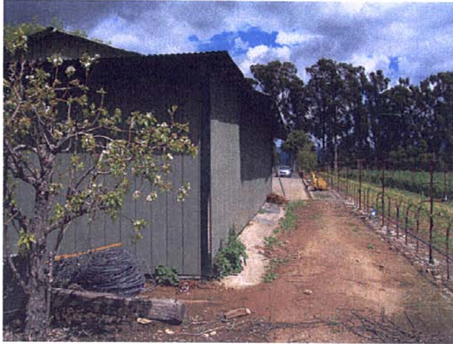
Photograph 1: Northeasterly panoramic view of existing barn, May 5, 2010
