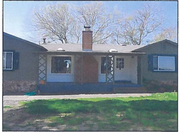
FIGURE 5: FRONT (NORTHEAST SIDE OF HOUSE).
