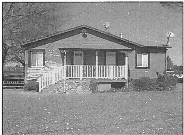
FIGURE 6: SOUTHEAST SIDE OF HOUSE. DETACHED GARAGE IS IMMEDIATELY TO THE LEFT OF THE PHOTO POINT.
