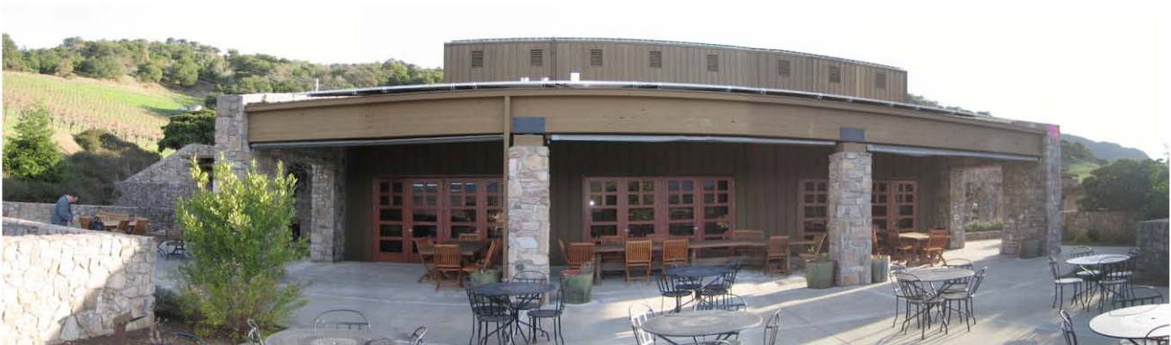
9. View of guest terrace looking Northeast; doors to office in background.
