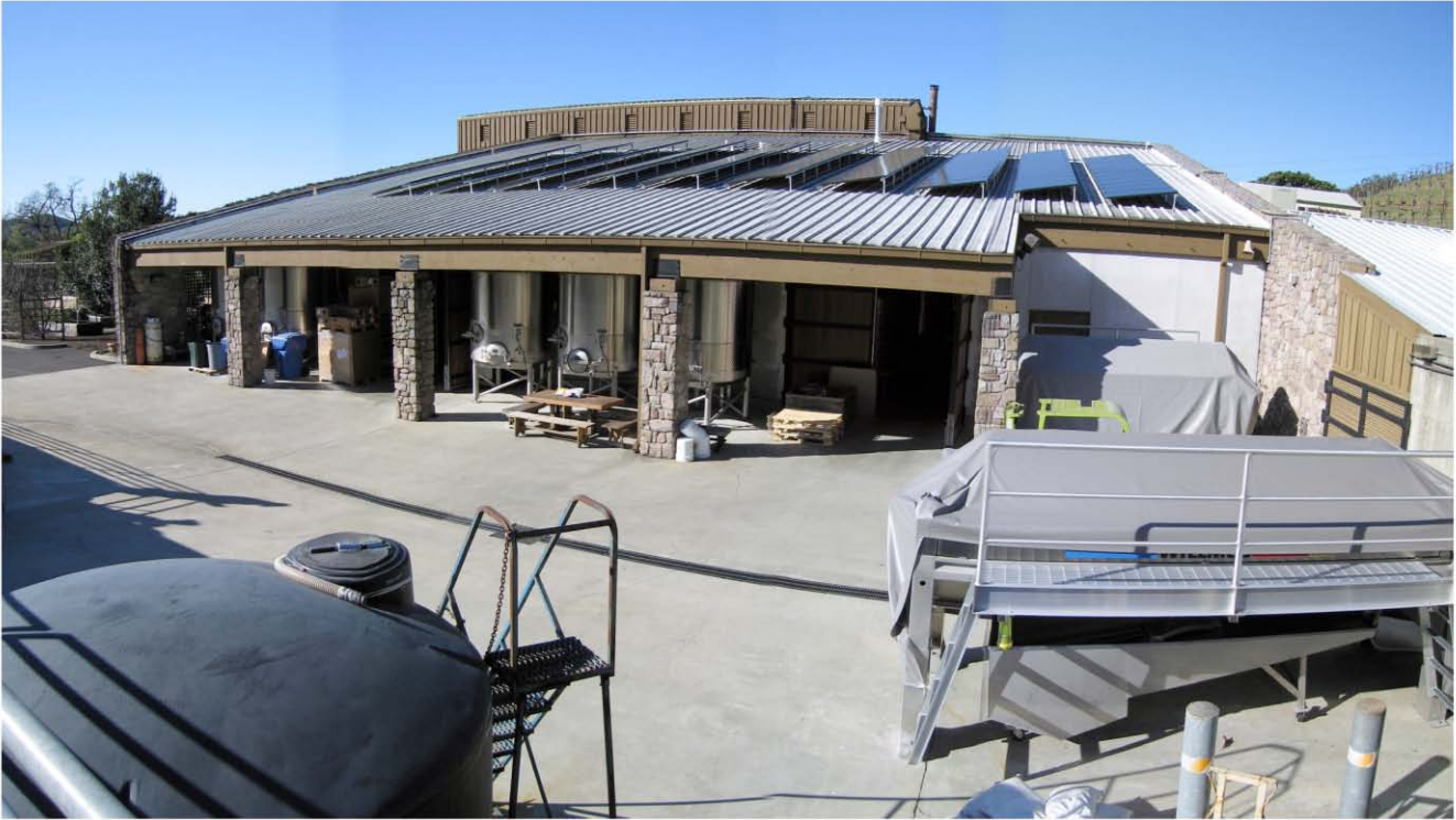
6. View of crush pad/production area looking Southwest. Edge of garden at far left, mechanical room at far right.
