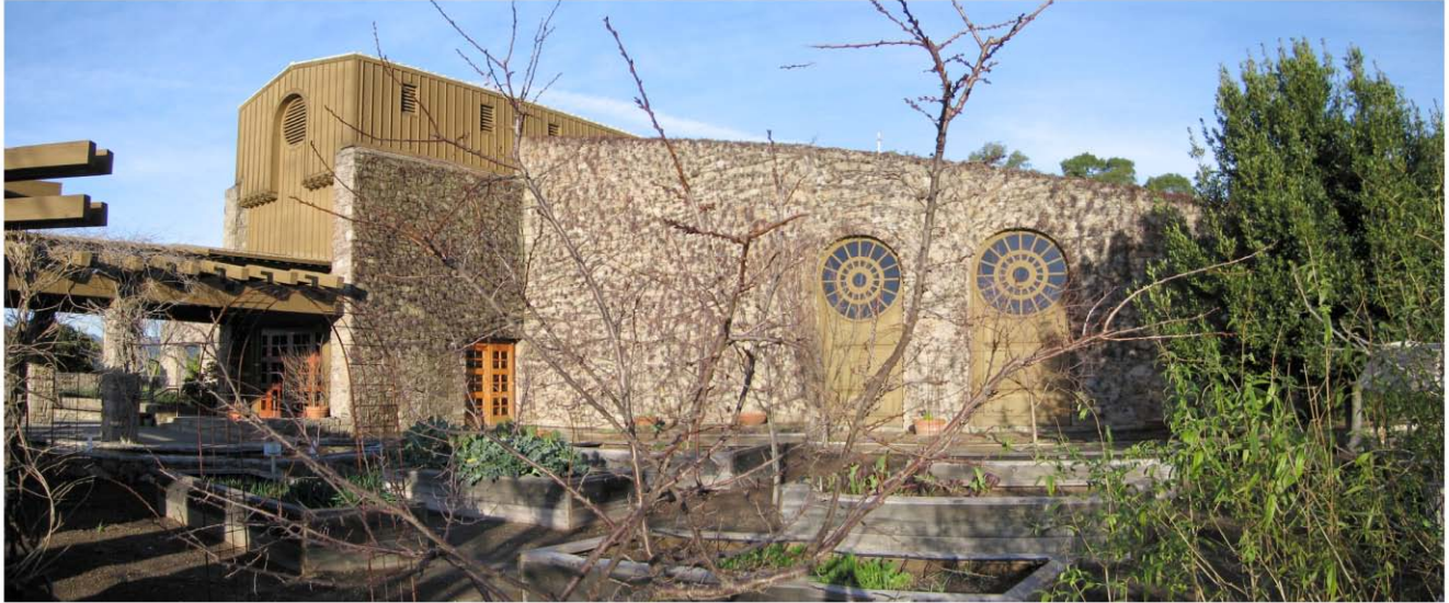
4. View of Main Entrance looking Northwest; garden in foreground.
