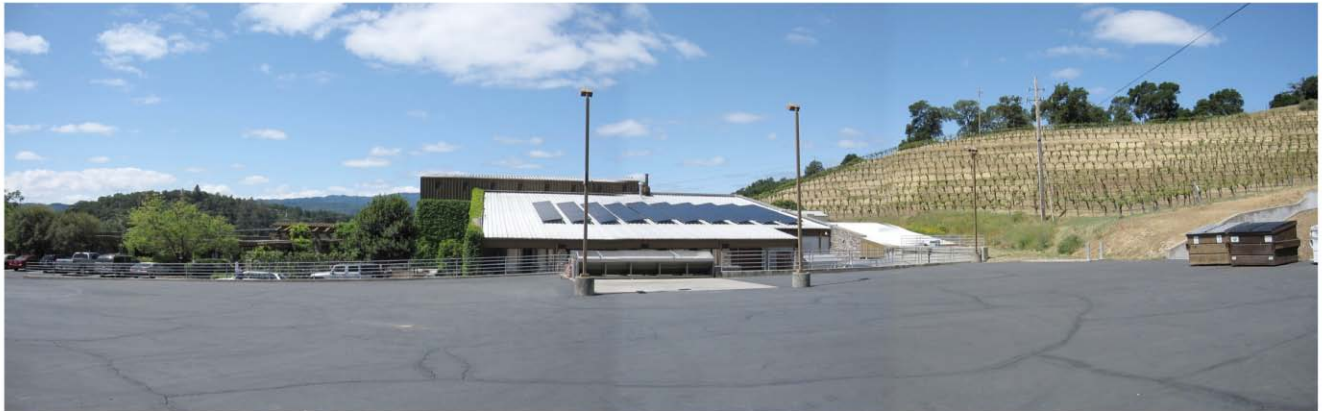
5. View of winery looking Southwest; production staging area in foreground, employee parking at left, cave entrance at far right.
