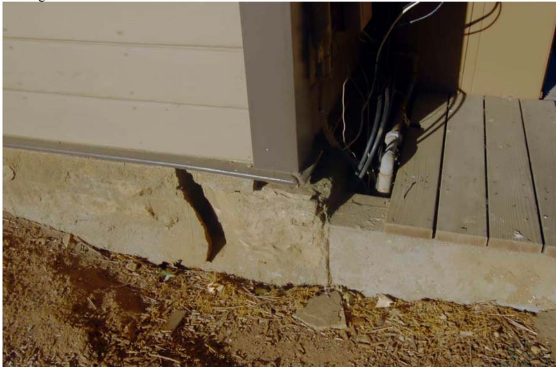
Carriage House foundation detail:
