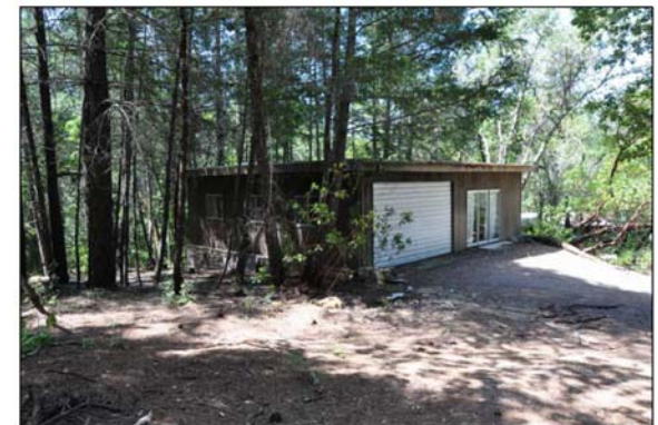
④b EXISTING GARAGE TO BE DEMOLISHED
