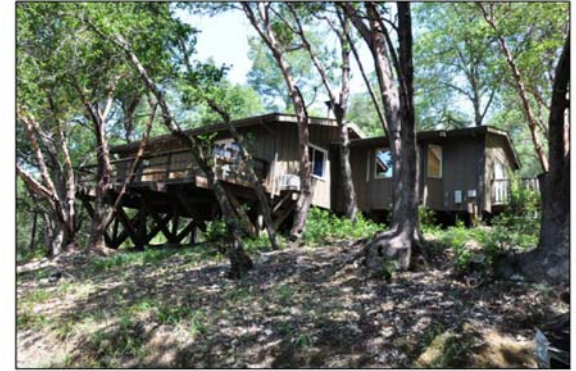
5b) LOOKING EAST ON DRIVEWAY AT EXISTING HOUSE
