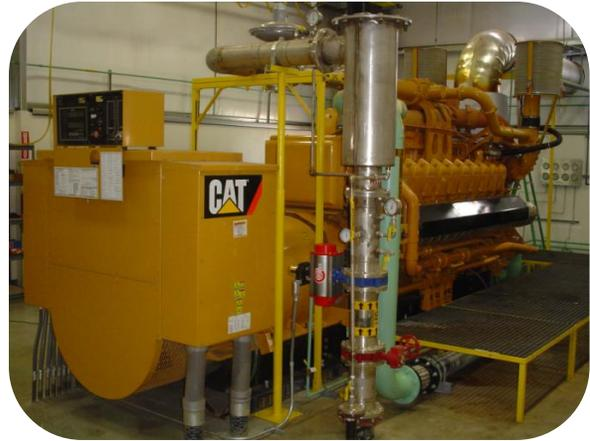
A similar facility is currently being constructed at the Recology Hay Road landfill. This plant will generate 1.6 MW of electrical power and has been designed for future expansion. Not only do these power plants convert greenhouse gasses into a renewable energy, they also serve as a best available control technology in minimizing emissions to the atmosphere.
