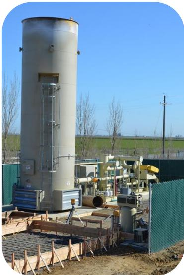
Recology Hay Road controls landfill gas (LFG) by utilizing an active LFG collection system connected to an enclosed landfill gas flare. The collection system includes 41 landfill gas wells and connection to the leachate collection and removal systems (LCRS). The enclosed flare has a maximum capacity of 1500 standard cubic feet per minute (scfm) and a minimum capacity of 150 scfm. The site currently collects about 600 scfm of landfill gas.
