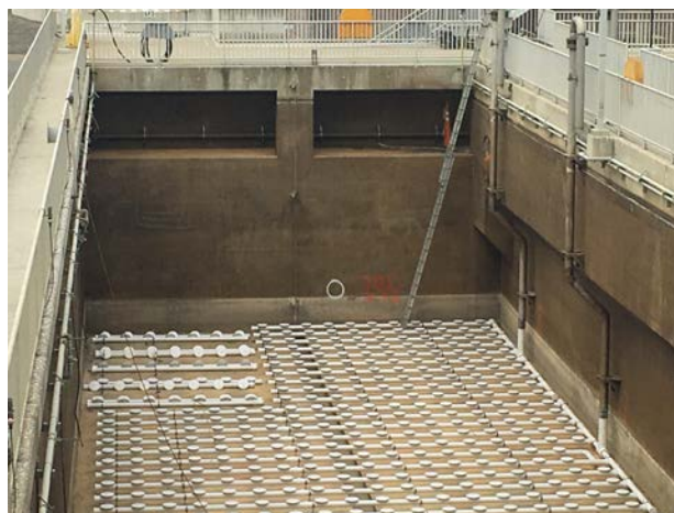
The aeration basin panels were replaced in 2017.
