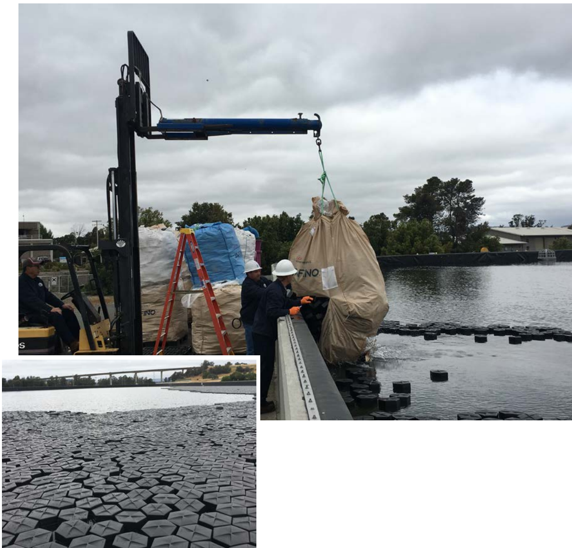
Installation of the floating covers on the recycled water reservoir at the Soscol Water Recycling Facility.
