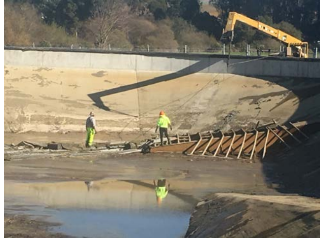
New recycled water reservoir liner installed in 2018.
