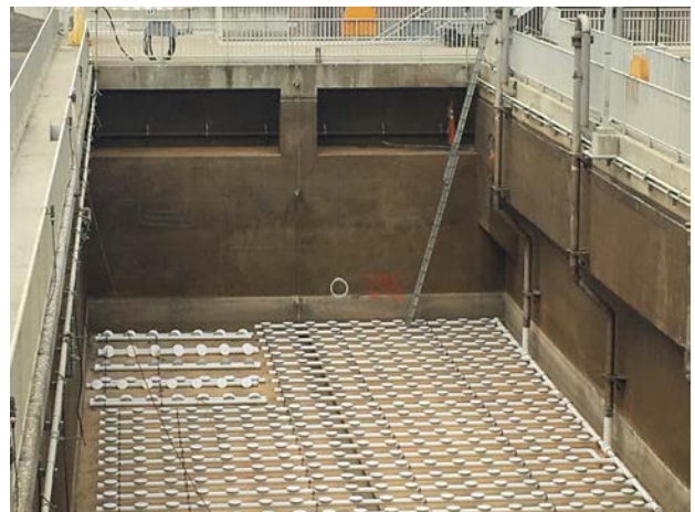
The aeration basin panels were replaced in 2017.
