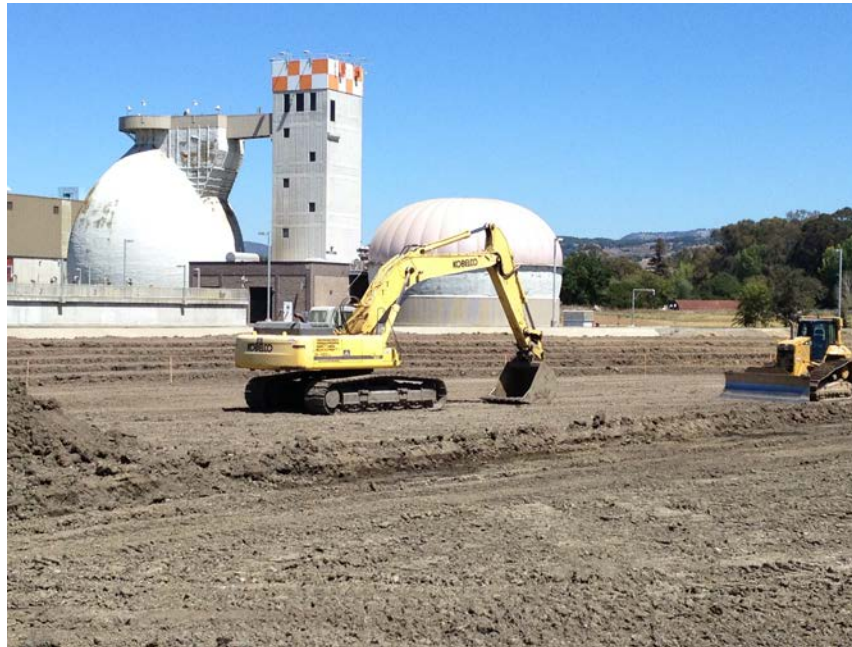
Construction of the secondary effluent equalization basin in 2014
