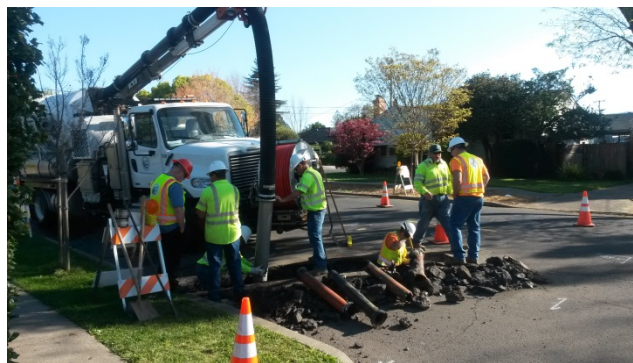
Collection system workers excavate a sewer lateral to make repairs
