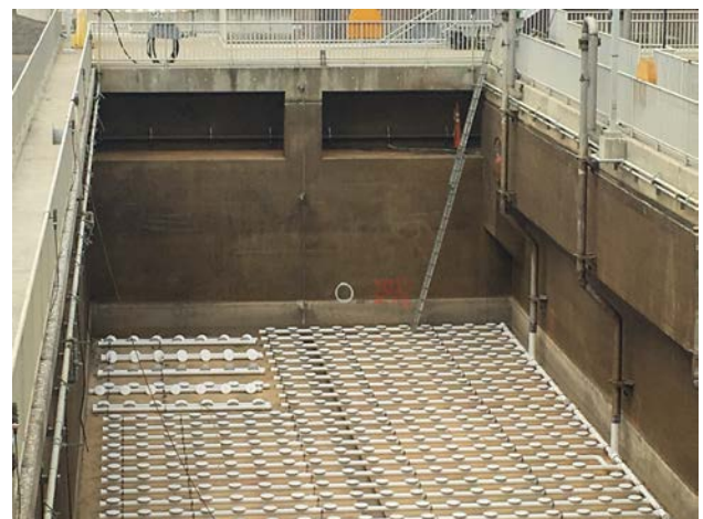
The aeration basin panels were replaced in 2017.
