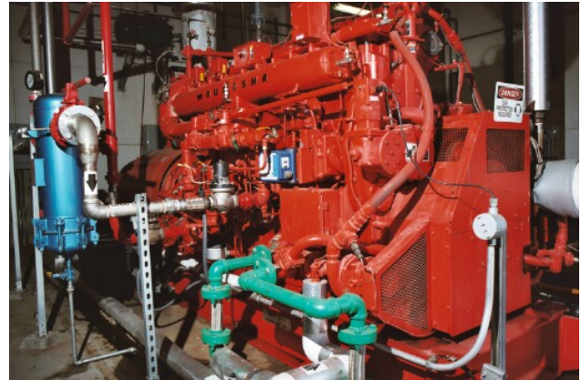
NapaSan's cogeneration engine burns biogas from the digester to create heat and electricity
