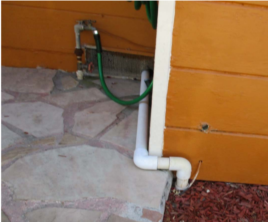
Sump pump pipe leading into the ground
