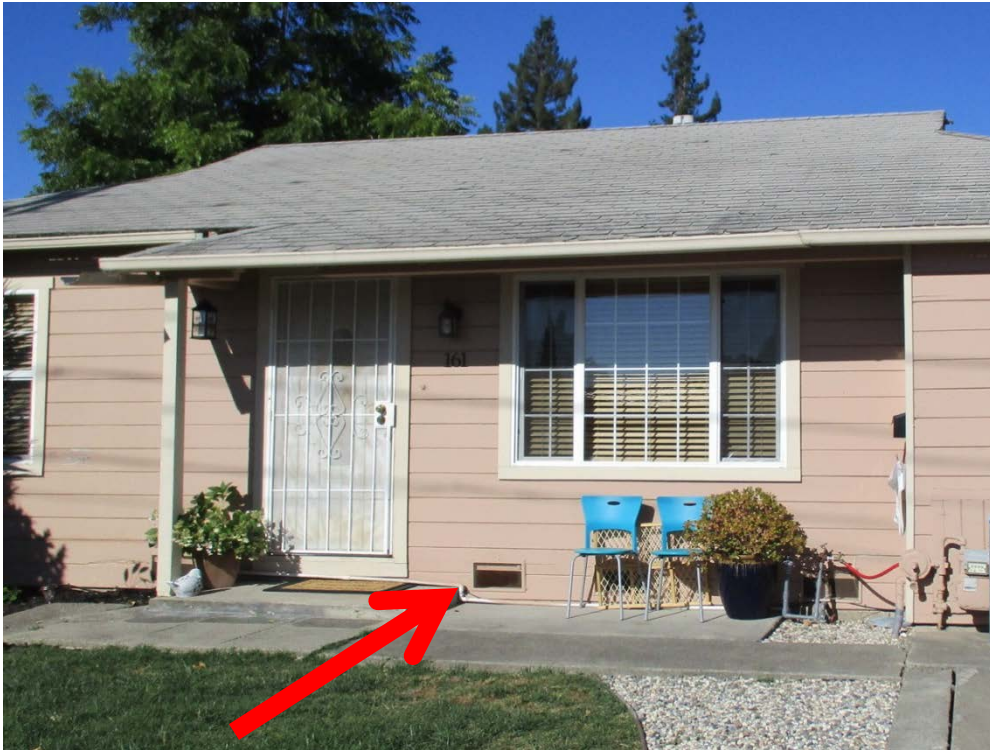
Raised-floor foundation and crawlspace
