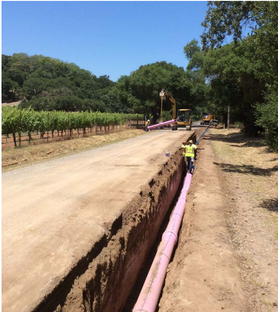
Installation of recycled water pipeline in the Los Carneros Water District area
