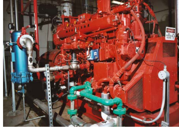
Cogeneration engine meets 40% of NSD's electricity from biogas.
