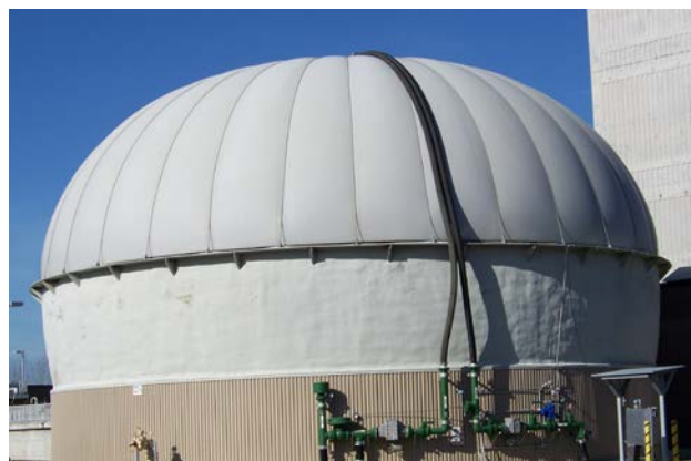
The Dystor cover, which serves as the biogas holder, was replaced in FY 2013/14 due to a rip in the inner membrane.
