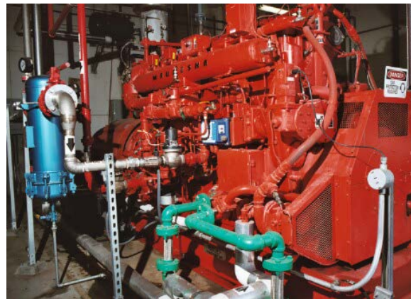
Cogeneration engine meets 40% of NSD's electricity from biogas.
