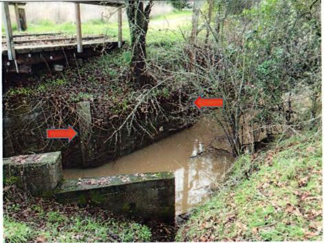
This 10 foot section of existing wall may remain, to provide necessary erosion scour protection. If it is deemed too weak to stand in place, it will be replaced with VRSS. Any replacement material will not exceed 1 cubic yard per running foot of stream. Avoidance of fill and in-stream construction activity will also void the need to acquire a Section 404 federal permit from USACOE.
