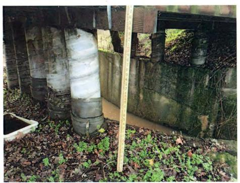
Concrete support posts and most concrete revetment walls will be lifted and removed from the bed and banks taking care not to allow rubble or detritus from entering the channel cross section as fill.
